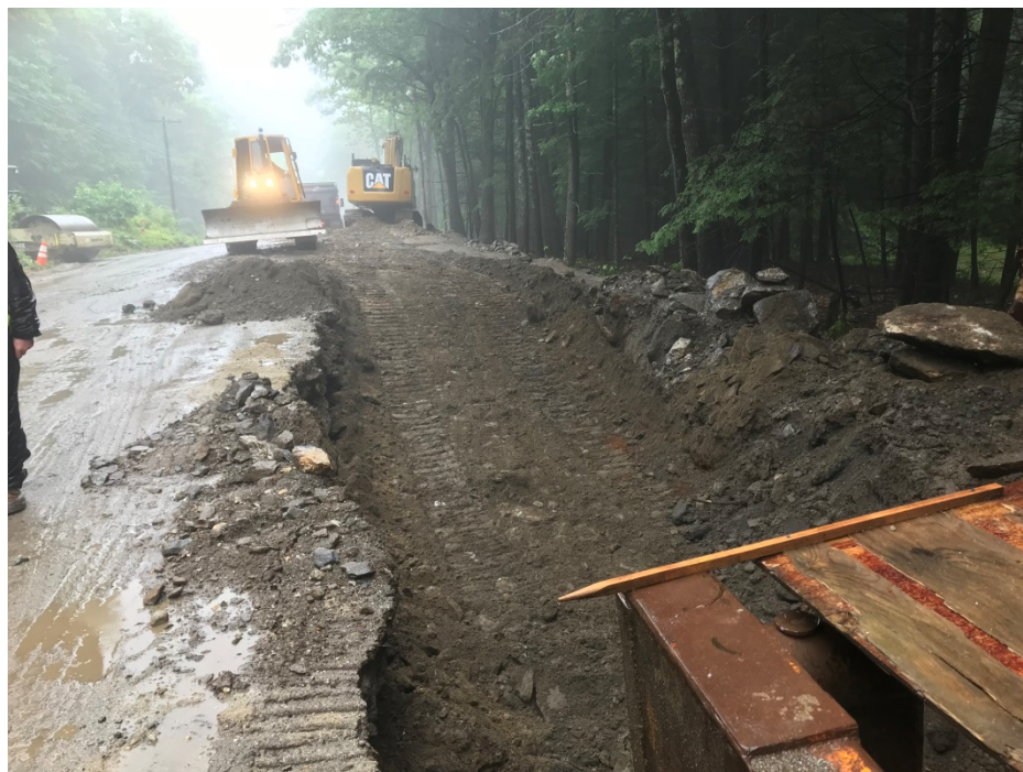
Photo 4 – Backfilling trench for water main near Tall Pines Way
