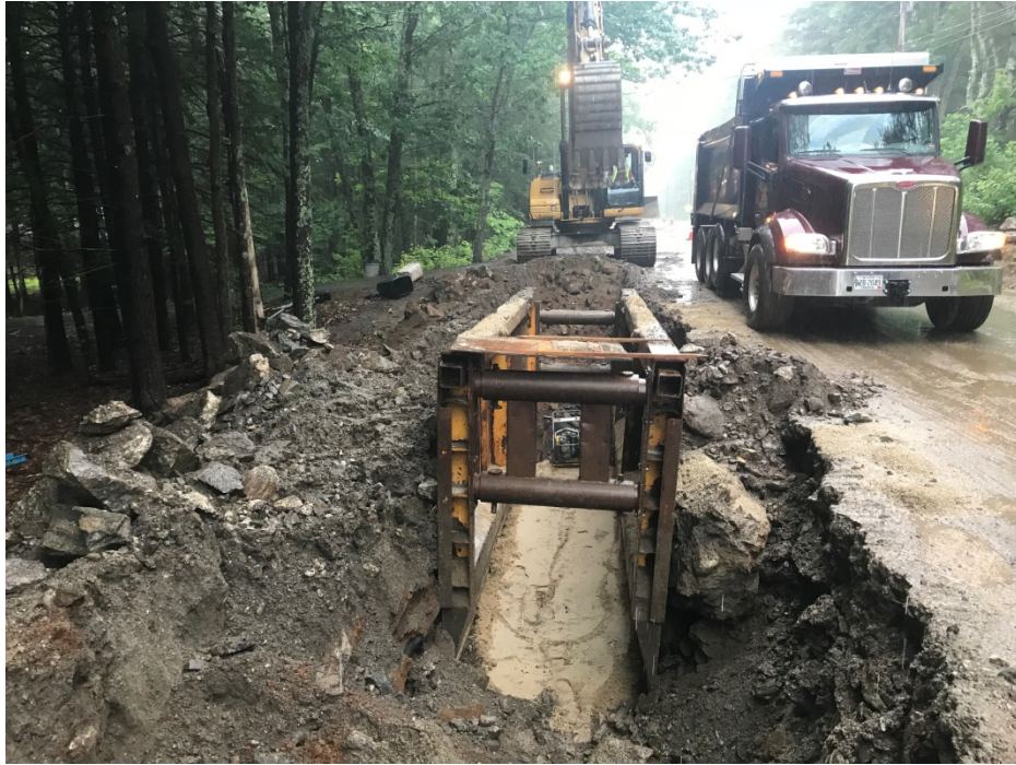
Photo 1 – 12 inch water main installed near Tall Pines Way
