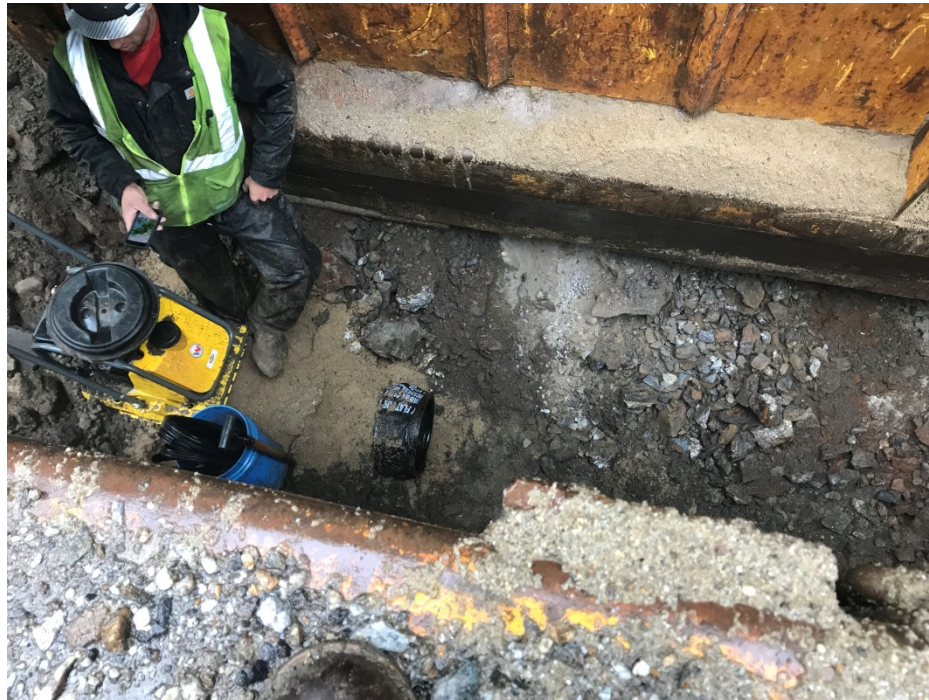
Photo 3 – Preparing bell end for 12 inch water main
