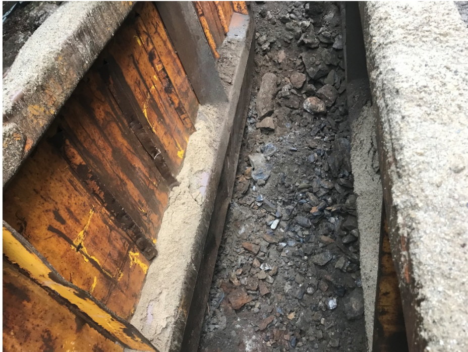
Photo 2 – Excavating trench for 12 inch water main near Tall Pines Way
