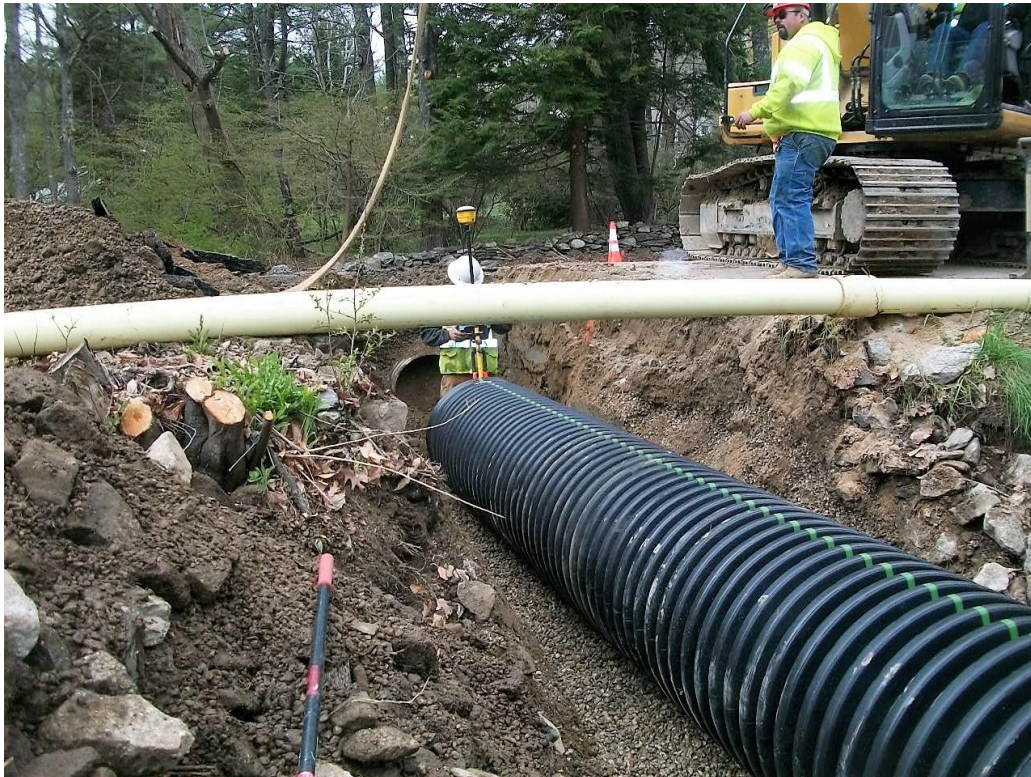
Downstream half of new 30" HDPE culvert installed over waterline.
