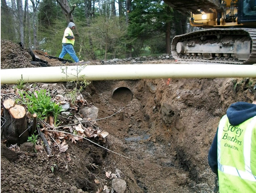
Upstream half of existing 24" HDPE culvert at STA 78+27 with 12" water main in the foreground.
