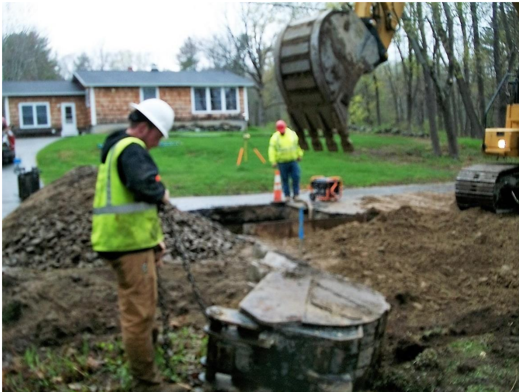
Preparing to remove ledge to install water service at 146 Middle Road
