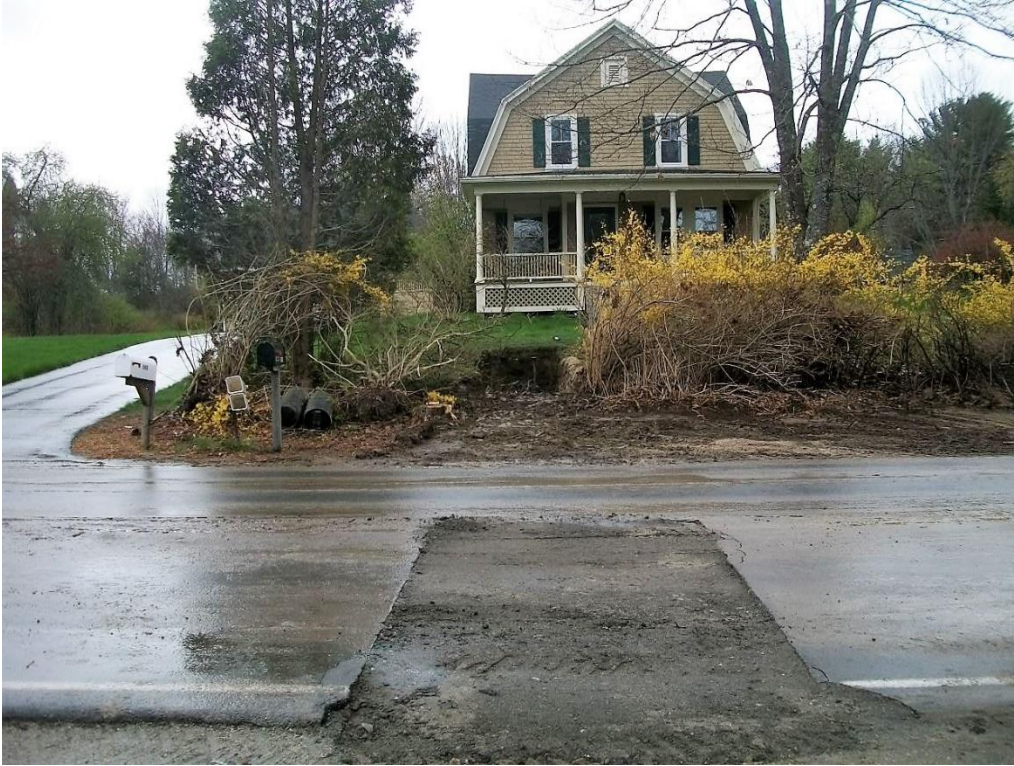
Water service installed at 142 Middle Road by pulling new line under road.
