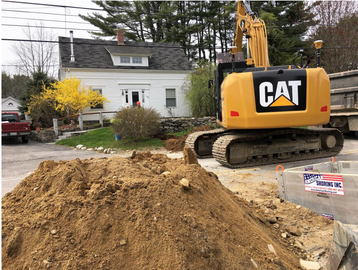
Preparing to pull replacement water service line under road.
