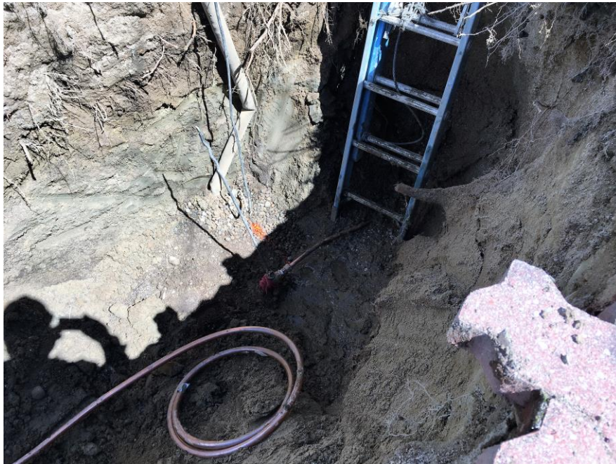
Connection of new "Curb Stop" valve from homeowner side of service to new 1-inch copper line to main.
