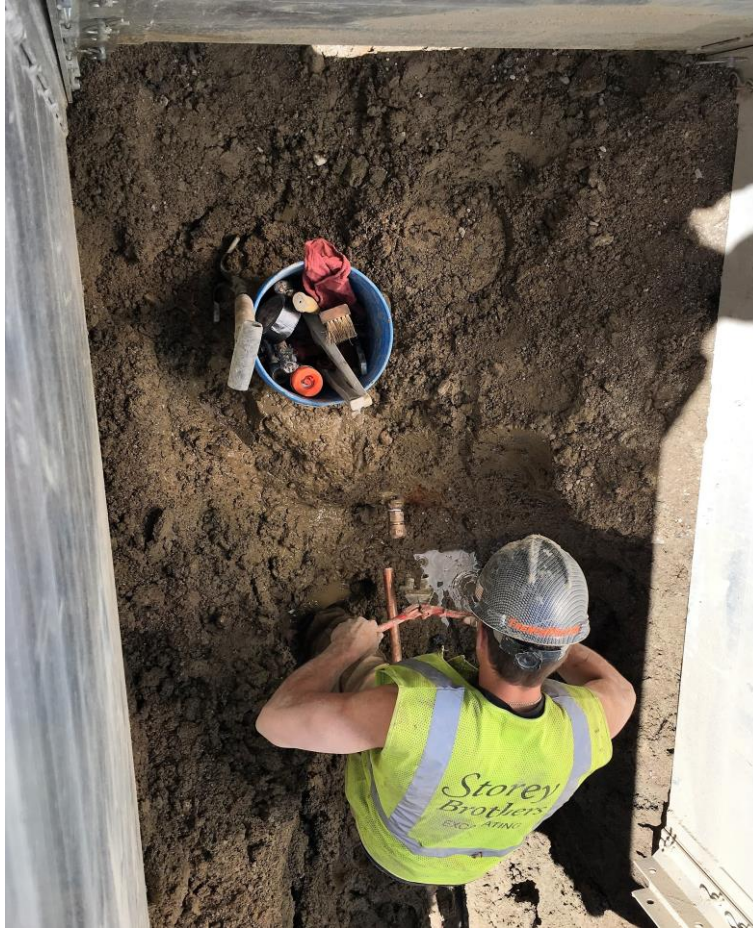
Connection of new service line to new "Corporation Stop" valve off the existing 12-inch water main.
