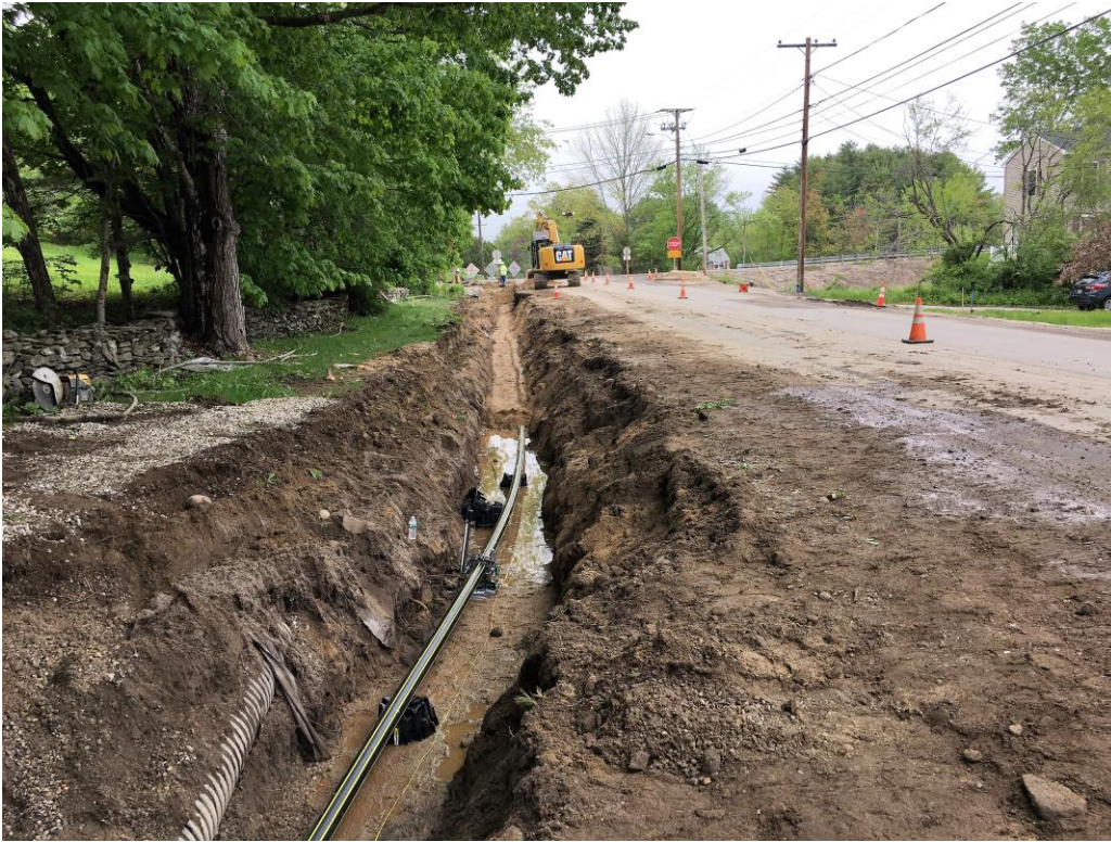
Initial fused segment of gas main placed in trench from Tuttle Road. Pre-existing 12-inch underdrain exposed on the left just north of catch basin CB-8B.
