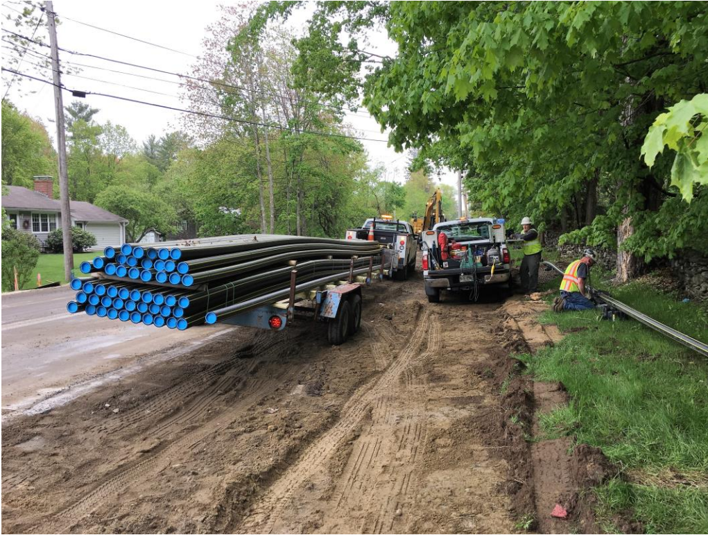
Summit crew welding initial sections of plastic pipe together prior to excavation of trench.
