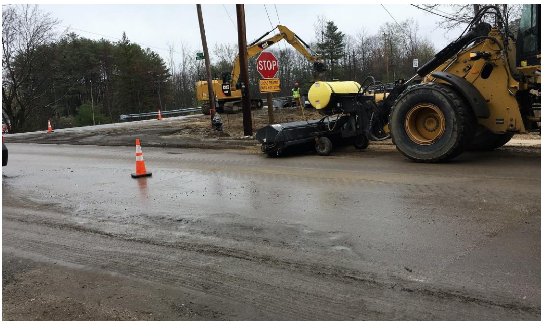
Cleaning up Middle/Tuttle connection area to resume work on renewing water services.
