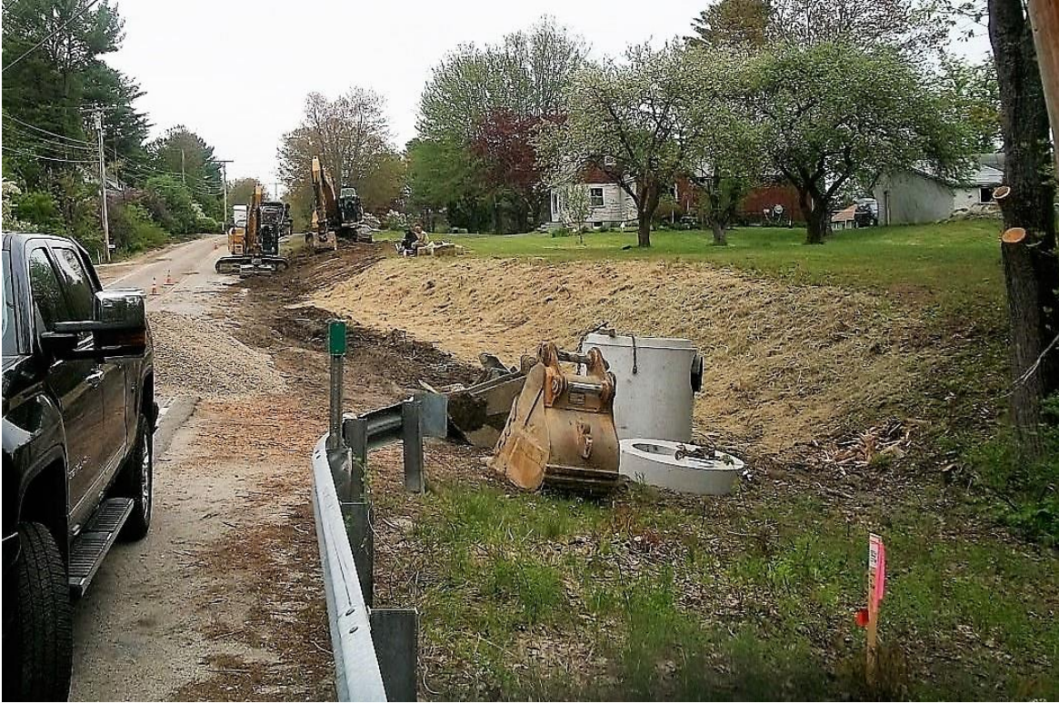
Stump removal and installation of geotextile reinforced slope at 117 Middle Road (Casey).
