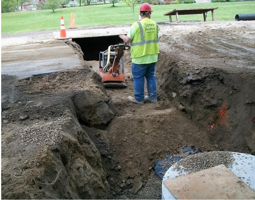
Sand placed from fabric over stone to subgrade of gravel and compacting prior to placing gravel to grade. CB-6E in foreground in front of 125 Middle Road.
