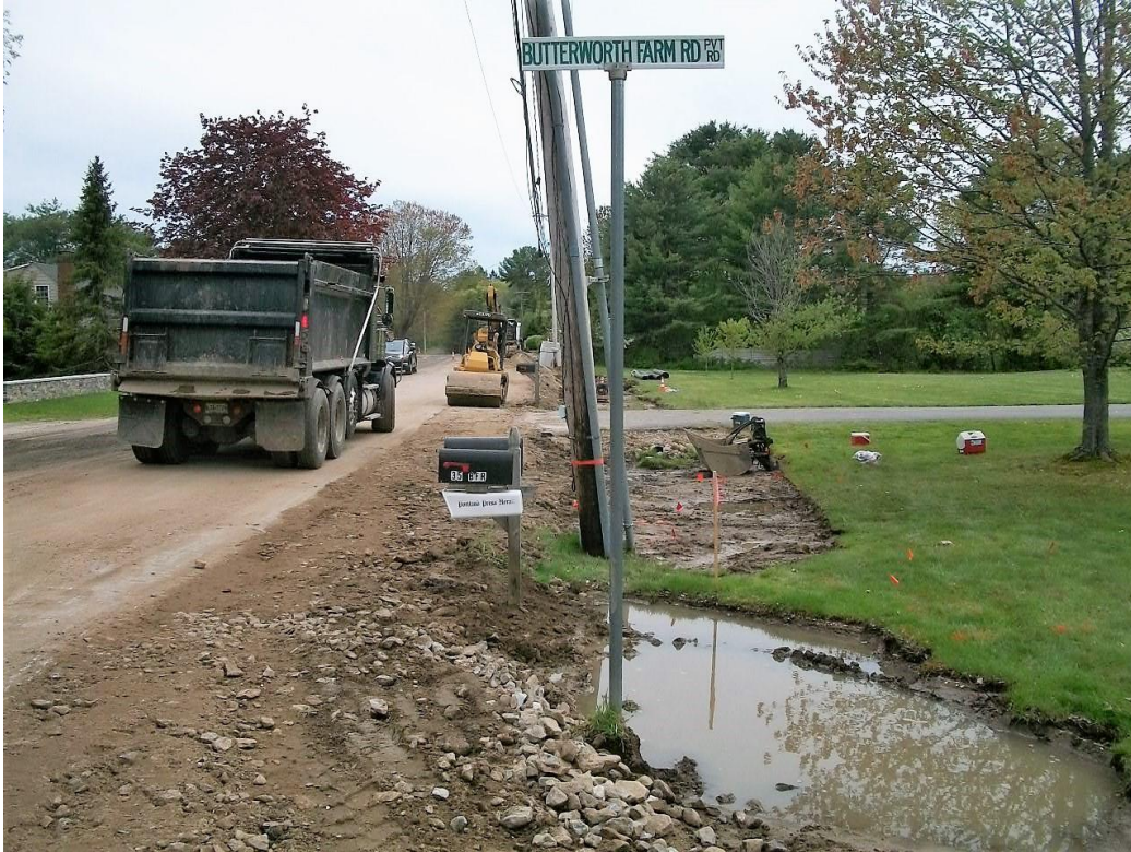
Compacted Type D gravel placed over crushed stone to grade behind underdrain installation.
