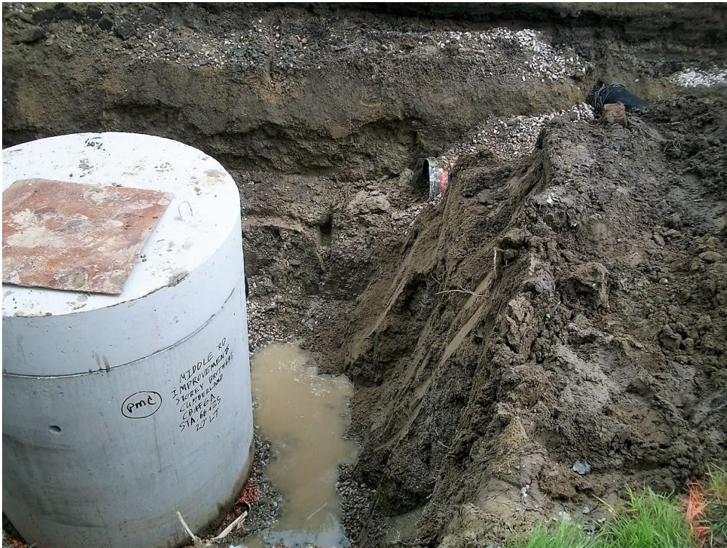
Catch Basin CB-6A installed per plan prior to connection to 12-inch underdrain outlet.
