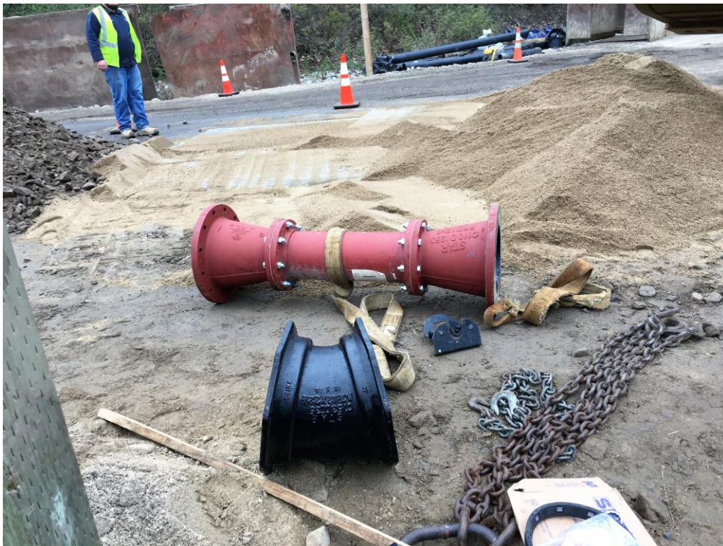
Spool & Reducer Assembly prior to being lifted into Vault.
