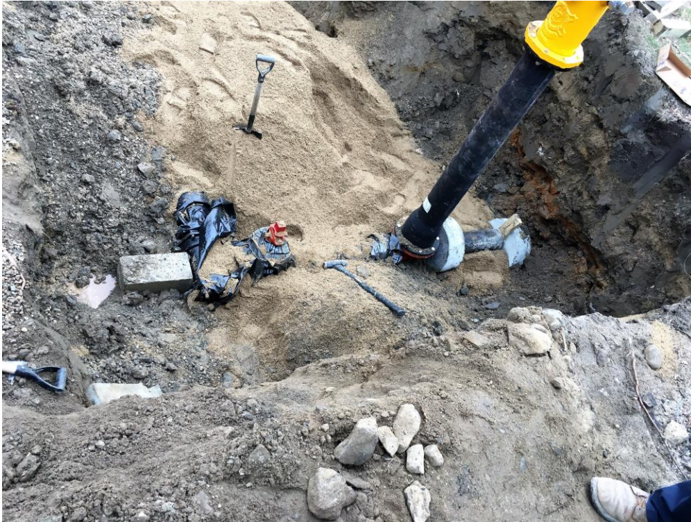
Hydrant assembly prior to final installation of thrust blocks and backfill.
