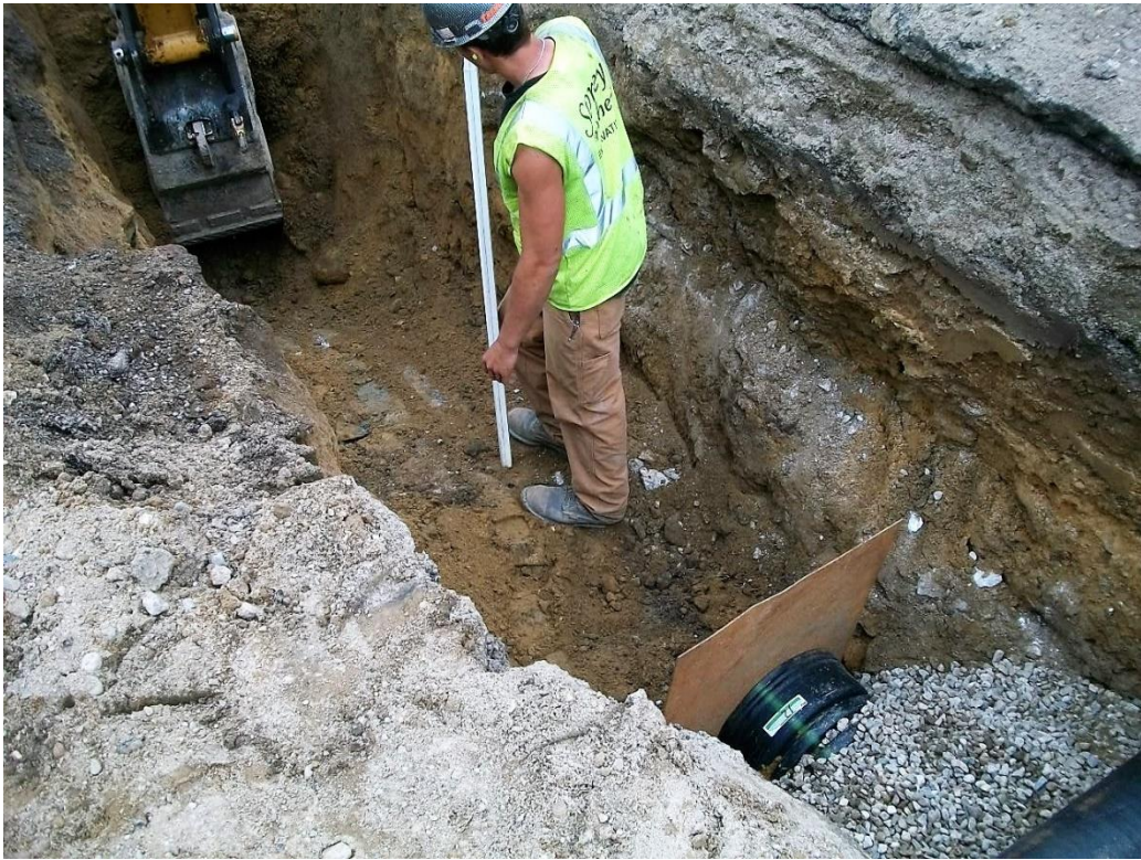
Estimating ledge to be removed during installation of 15" underdrain at driveway of 122 Middle.
