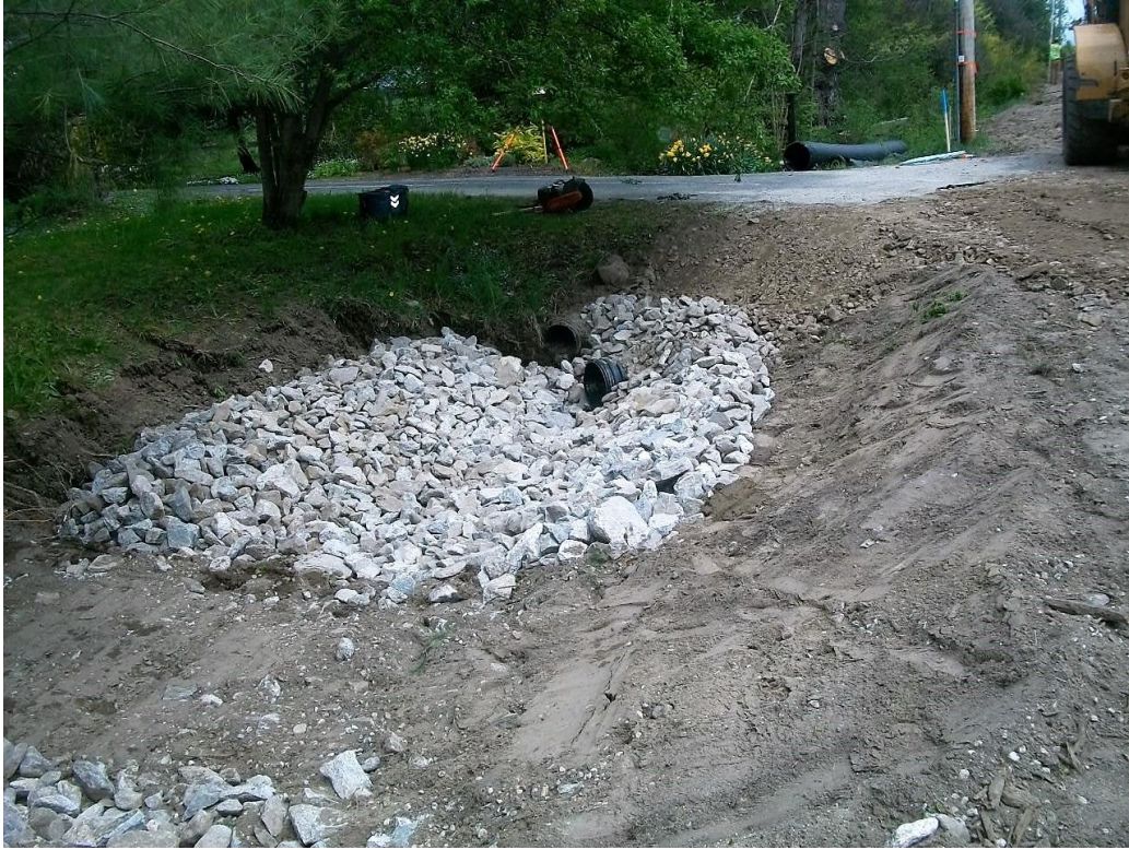
Outlet of 15-inch underdrain south of driveway for 116 Middle Road near STA 58+65.
