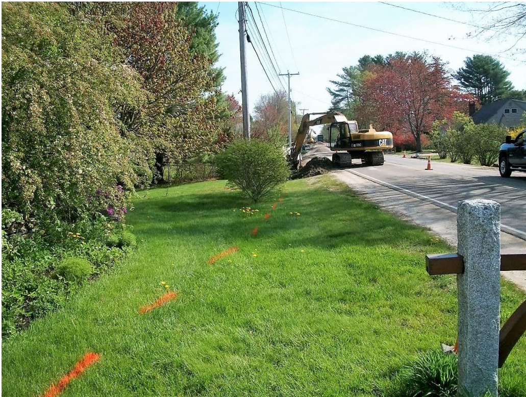
Stripping and rough grading drainage swale ahead of underdrain installation near STA 62+00. Proposed limits of construction painted in orange.
