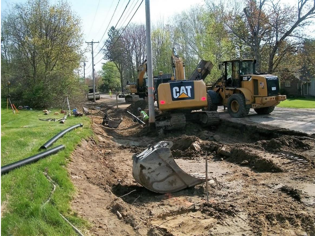
Resuming the installation of 6-inch underdrain to terminate at stake in foreground at STA 68+80.
