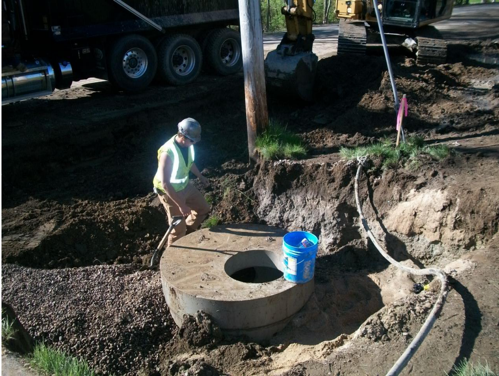
Resuming the installation of 12-inch underdrain from catch basin CB-7B at STA 71+55.
