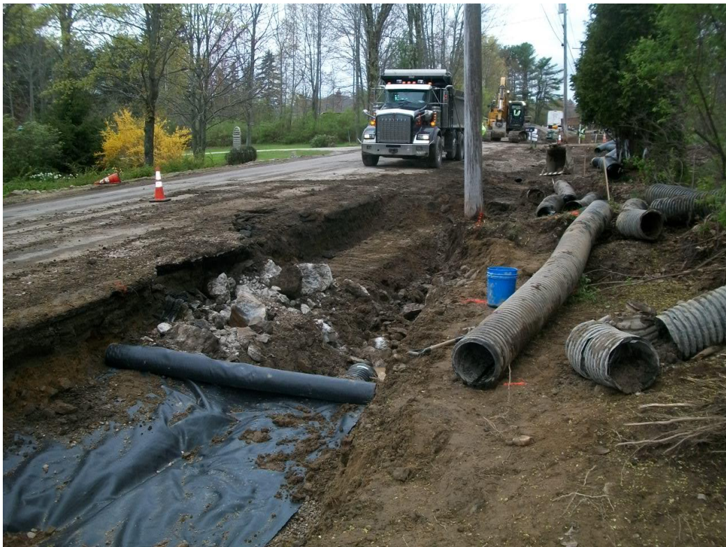
Ledge removal required in road subgrade at STA 73+10 between 142 & 146 Middle
