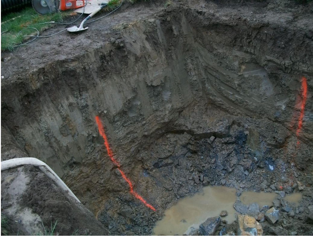
Ledge removal required to install catch basin CB-7B in front of 142 Middle.
