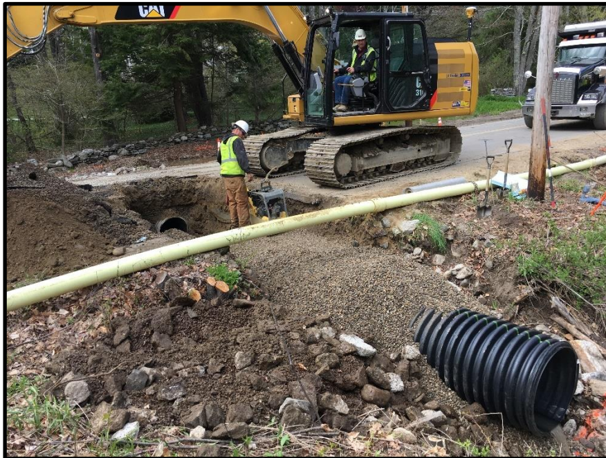
Photograph 4: Downstream half of new 30-inch HDPE culvert installed over waterline.
