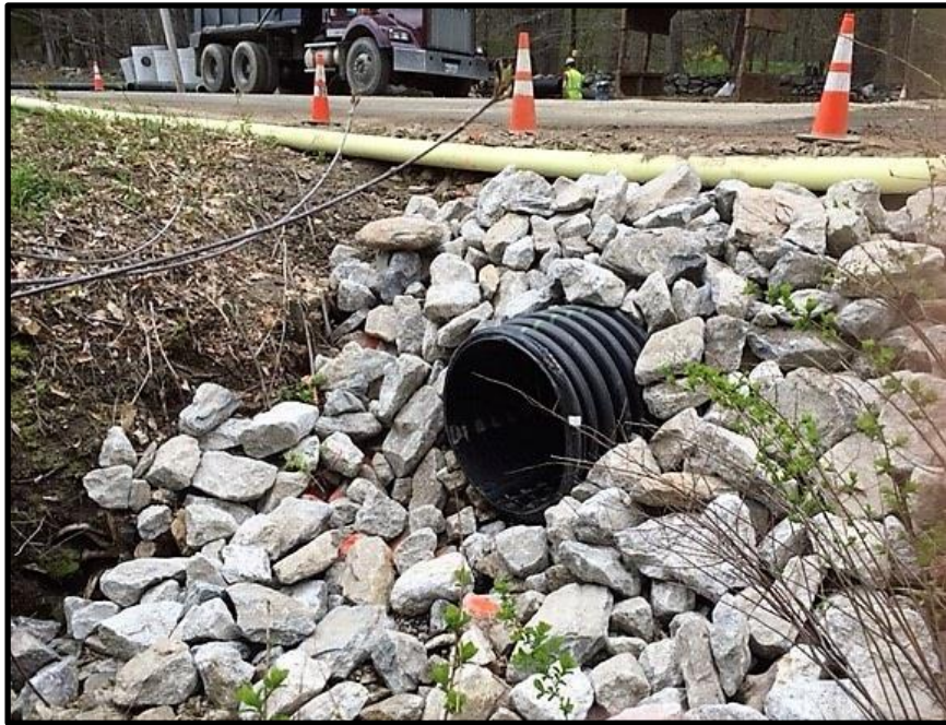
Photograph 5: 30-inch diameter HDPE culvert at outlet near STA 78+27.
