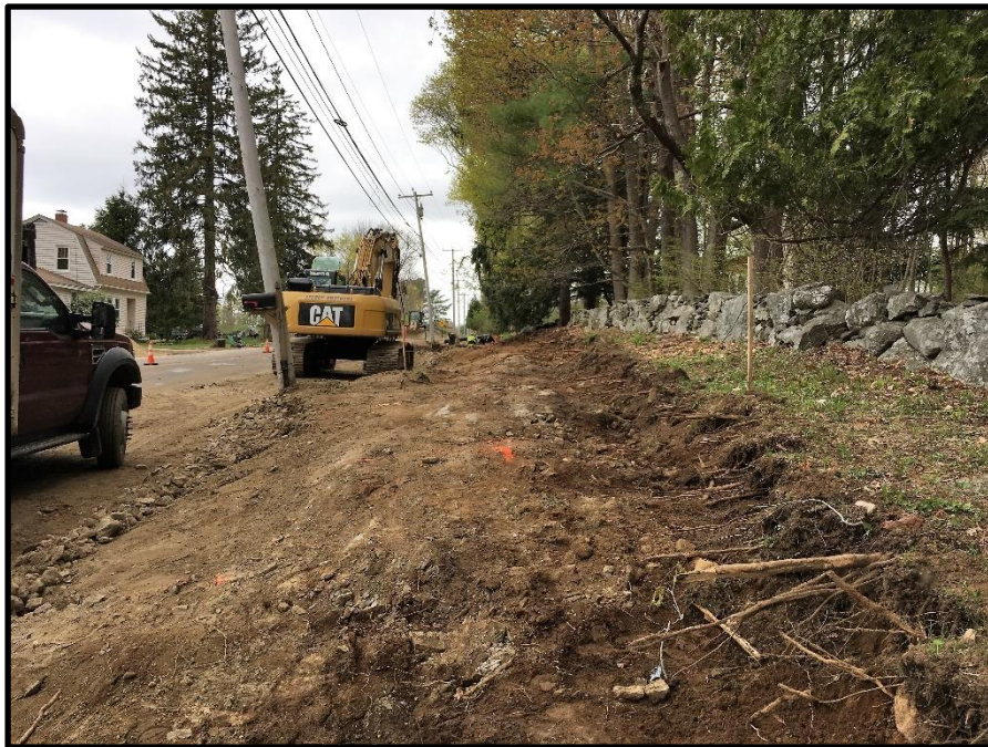
Photograph 10: Ledge exposed near STA 75+00 across from 147 Middle Road on back slope of swale
