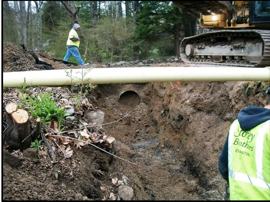
Photograph 3: Upstream half of existing 24-inch HDPE culvert at STA 78+27 with existing 12-inch water main in foreground.
