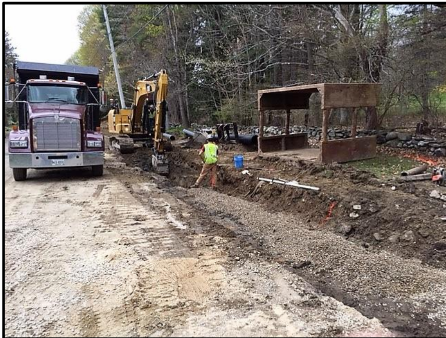
Photograph 6: Installation of 15-inch underdrain upstream of CB-7E.
