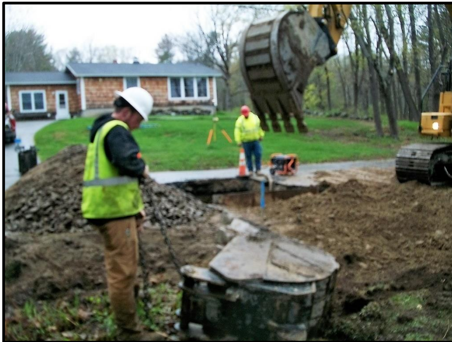
Photograph 2: Preparing to remove ledge to install service at 146 Middle Road.
