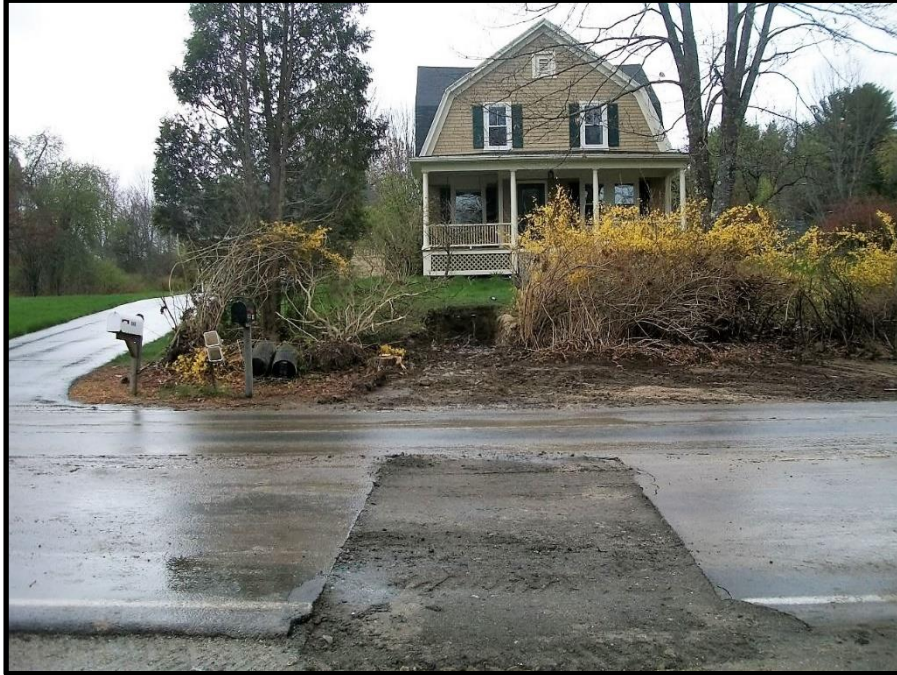
Photograph 1: Water service installed at 142 Middle Road by pulling new line under road.
