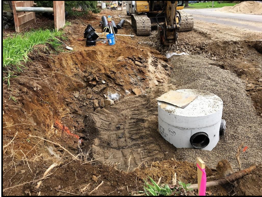
Photograph 9: Structure for Catch Basin CB-7C installed nearly entirely in ledge.
