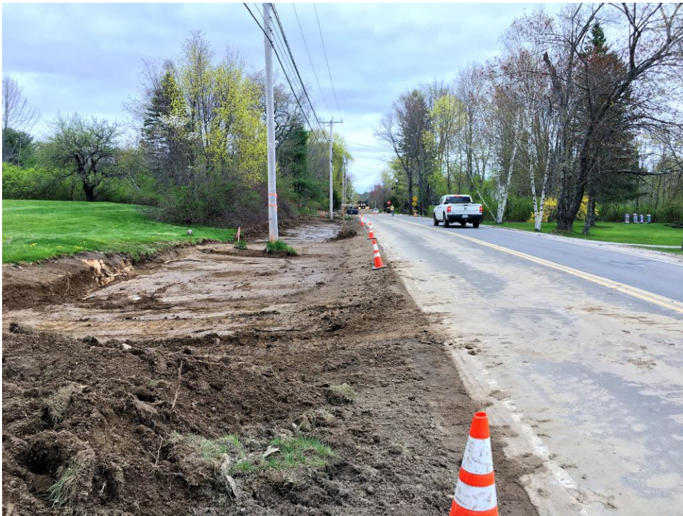
Grubbing and rough grading west side of road from Butterworth Farm looking northward.
