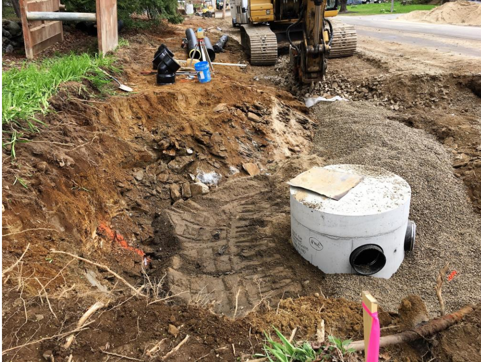
Structure for Catch Basin CB- 7C installed nearly entirely in ledge.
