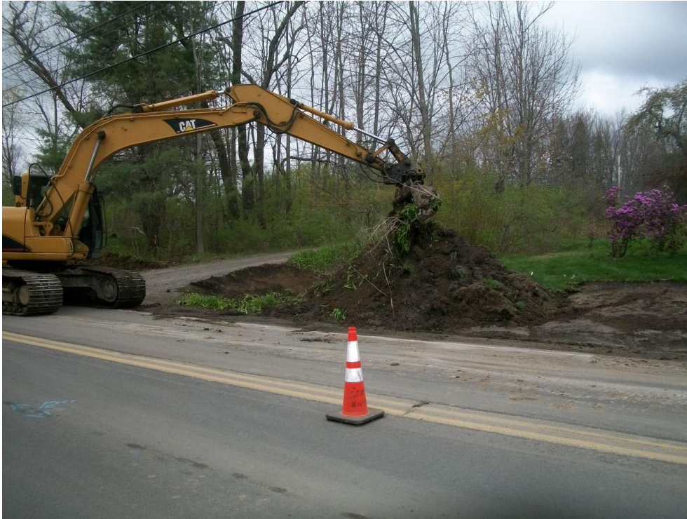
Additional excavator used to strip and rough grade the shallow drainage swales along west side of road between 140 & 142 Middle Road
