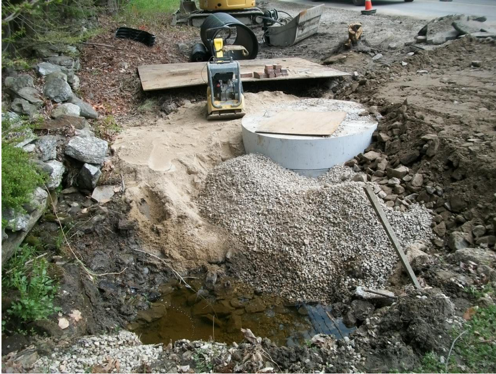
Structure for Catch Basin CB- 7E installed late the previous day was raised so 36" outlet could clear over the existing water main.
