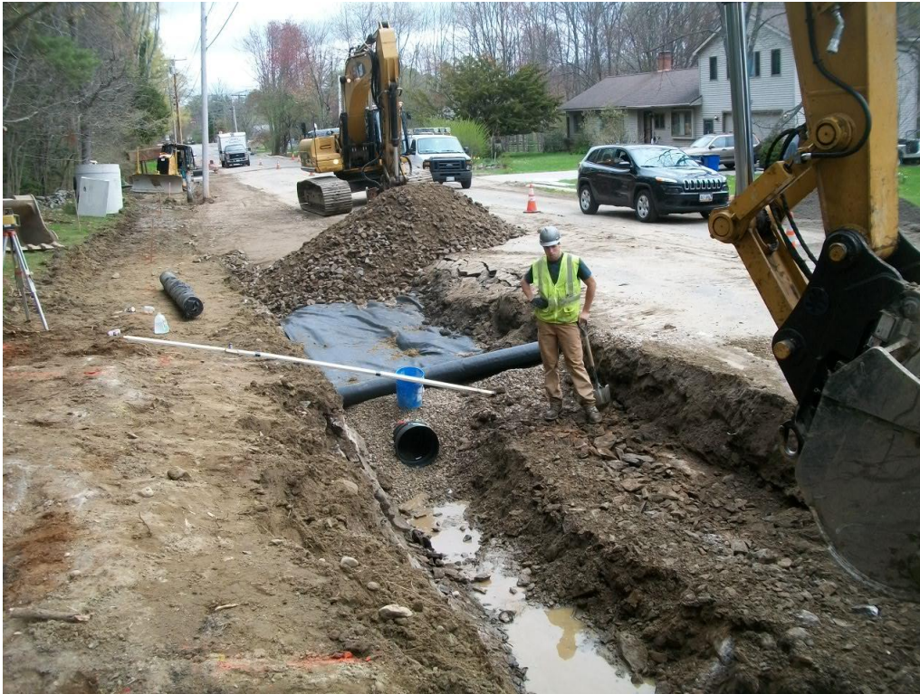
15-inch underdrain near STA 77+50 installed from CB-7E upwards towards CB-7C.
