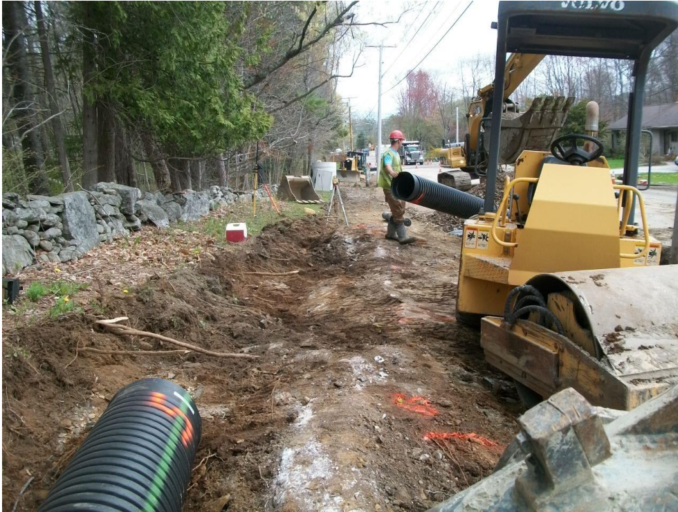
Ledge exposed after stripping away topsoil while construction of the back slopes of the shallow swales between CB-7E and CB-7C.
