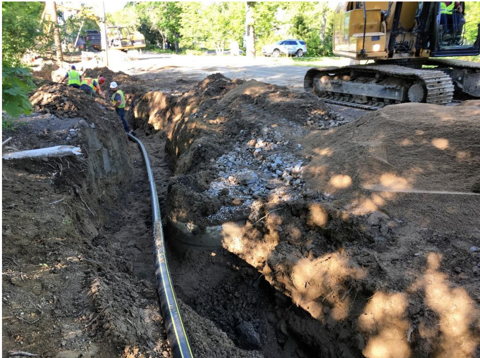
End of day of gas line installation from STA 71+75 looking back towards Pole 333. Gas line trenched behind catch basin CB-7A in front of Lewis driveway (140 Middle).
