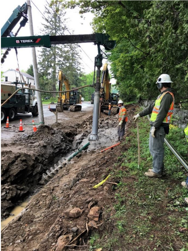
Coordination of drilling hole for Pole 336 through ledge with ledge removal & excavation of gas line trench.
