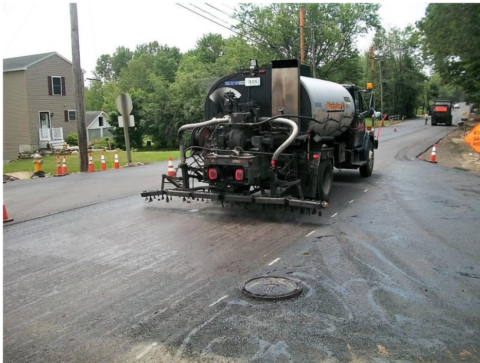
Tack truck spraying the pavement surface prior to placing the 2 nd layer of pavement.
