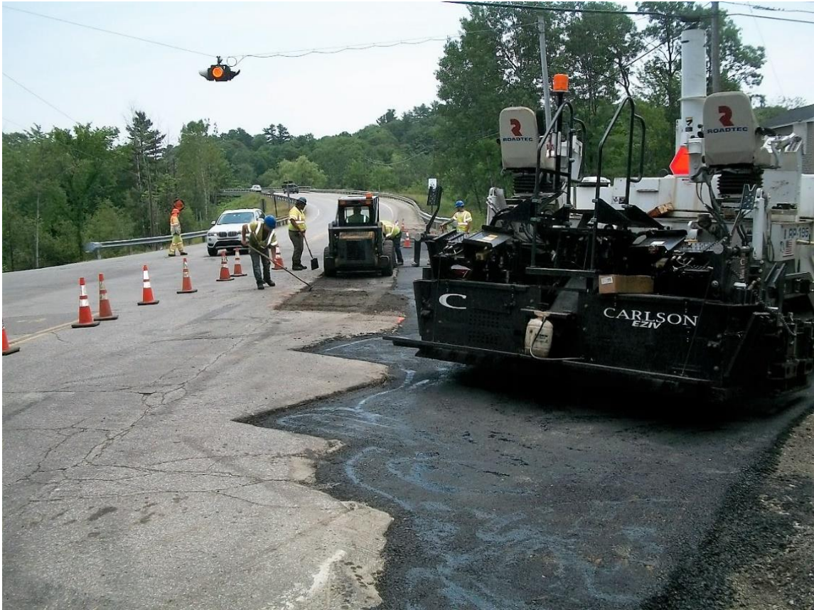
Cleaning up the temporary butt joint prior to placing pavement.
