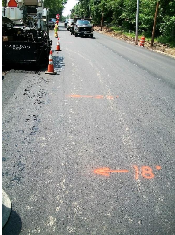
Layout markings prior to placing 2 nd layer of base pavement.
