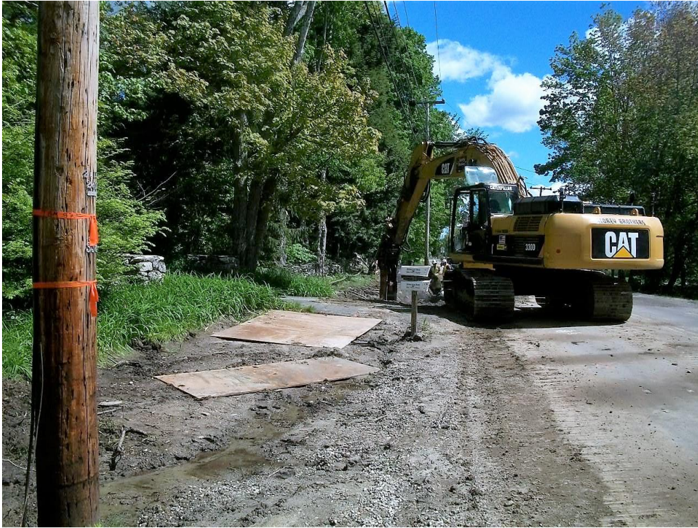
Using hoe ram to break up ledge at STA 79+50 just north of 158 Middle Road driveway (Knowles). Pole 338 in the foreground.
