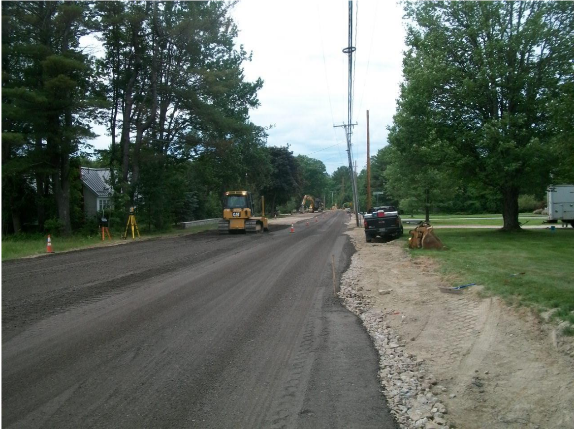
Placing millings on east side of road in a southerly direction near Butterworth Farm Road.
