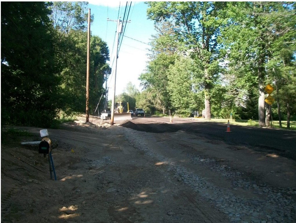
Placed reclaimed pavement millings in the afternoon from 146 Middle Rd. to 137 Middle Rd.
