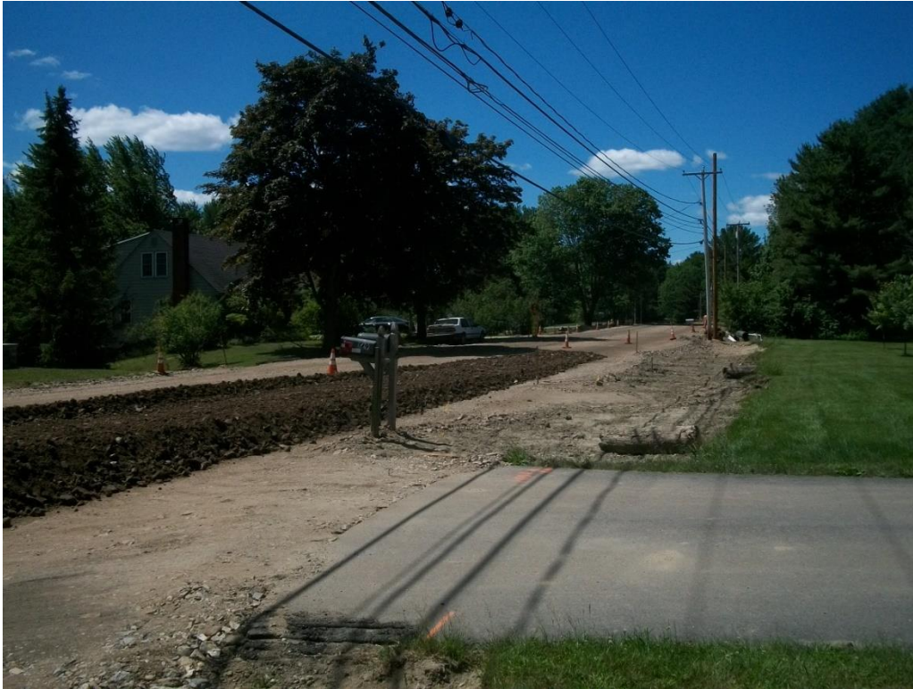
Placed additional Type D gravel in the morning from 140 Middle Rd. to 126 Middle Rd.
