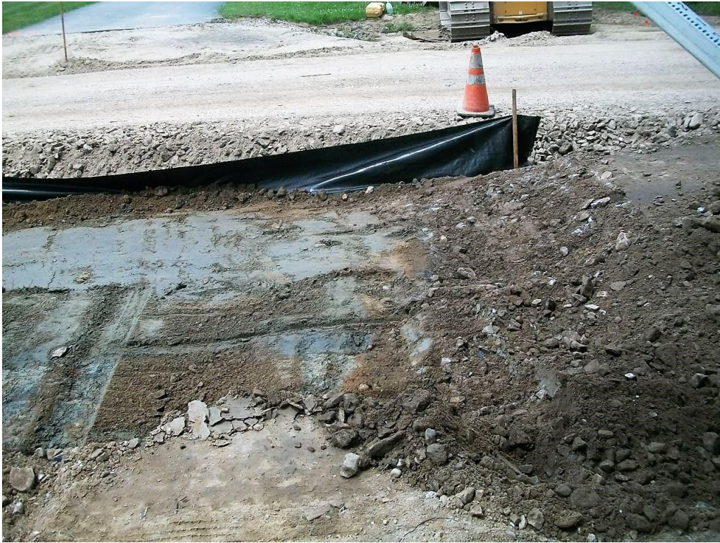
Subgrade of bluish gray clay at the driveway for 129 Middle Road was typical.
