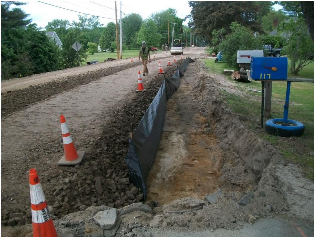
View at end of day looking north from the Casey driveway. Eastern edge of the road remained open so the remaining underdrain can be installed.
