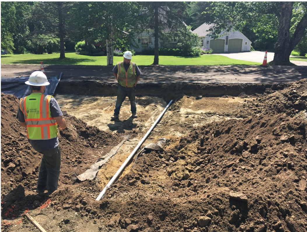
Summit crew placing PVC conduit sleeve for future natural gas service to 137 Middle Road under silty clay subgrade of road prior to backfilling.
