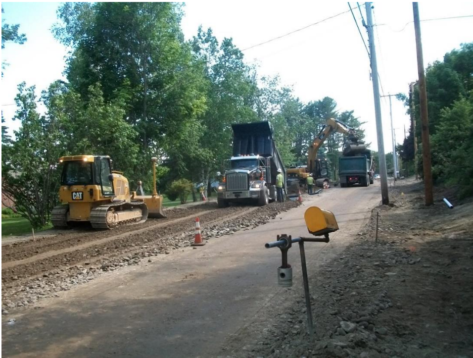
Excavating the eastern side of the road near the end of the day followed closely by placement of gravel. 140 Middle Road (Lewis) mailbox in foreground.
