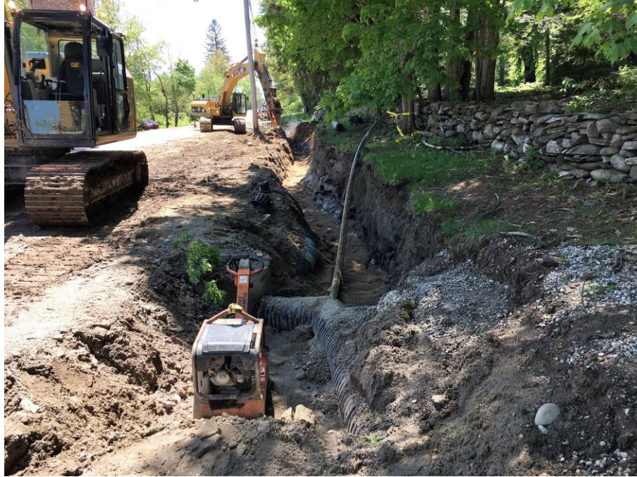
Trench excavated and sand bed placed but progress slowed by ledge removal using a hoe ram (background). Catch Basin CB-8B in foreground.
