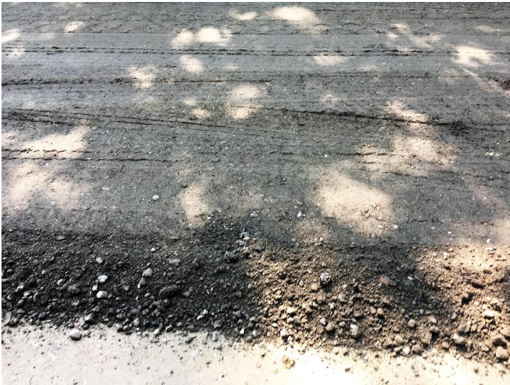
Close-up of reclaimed pavement used as surface gravel in lieu of Type A gravel.
