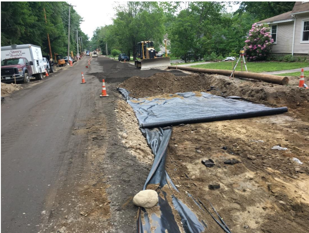
Excavation to subgrade then placement of fabric, Type D Base Gravel, and reclaimed pavement.
