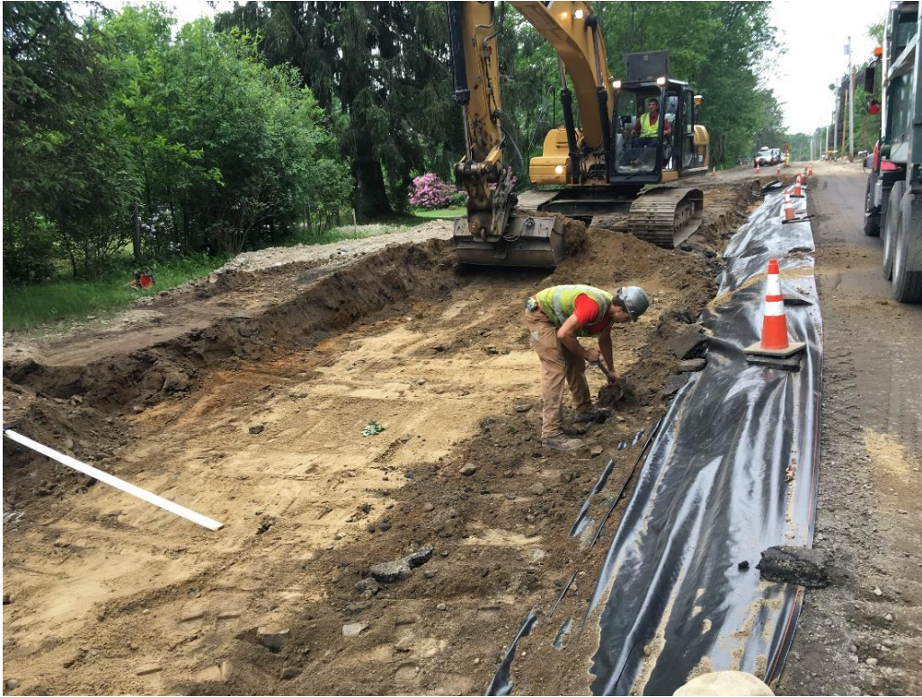
Improved subgrade conditions (less clay) along this segment of road.
