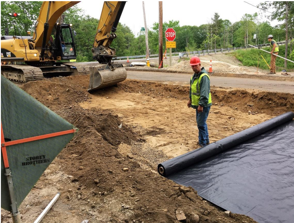
Less clay and much firmer subgrade approaching Tuttle road at STA 83+00.
