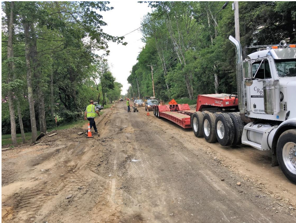
Northern section of the work zone near Tuttle Road where all the pavement was removed is very rough and needs to be touched up before restoring 2-way traffic for the evening.
