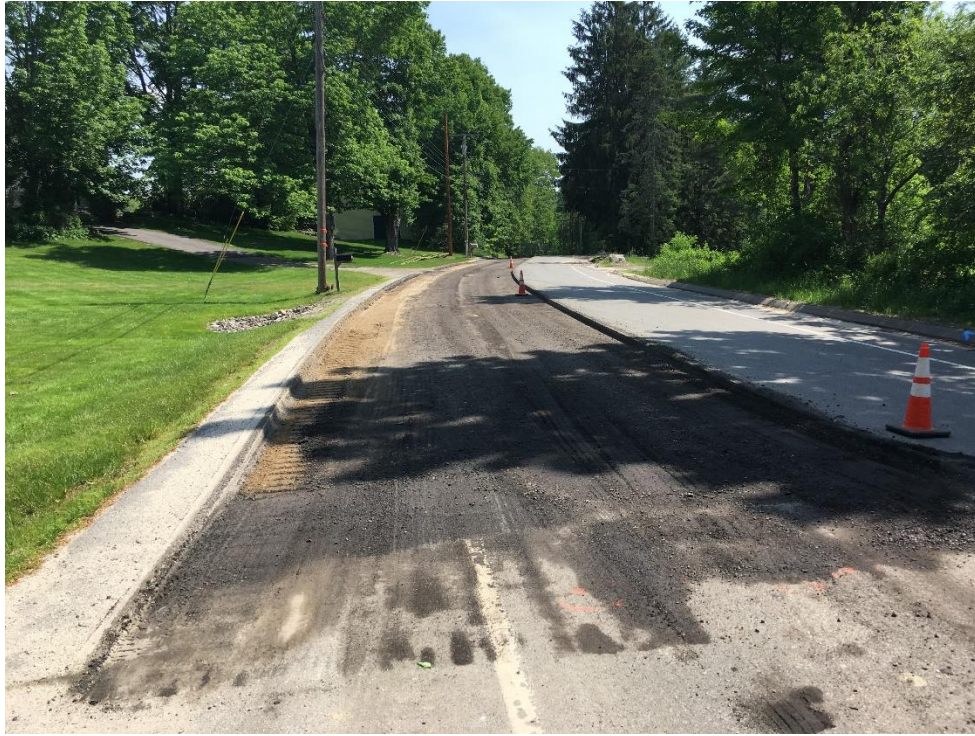
First 4-inch pass milling western side of road to the southern limit of the work zone across from 97 Middle Road.
