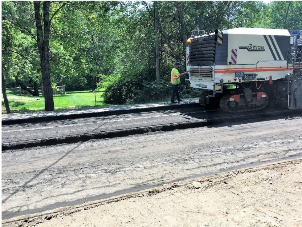
First 4-inch pass milling eastern side of road after 2 pass deep on western side (foreground)
