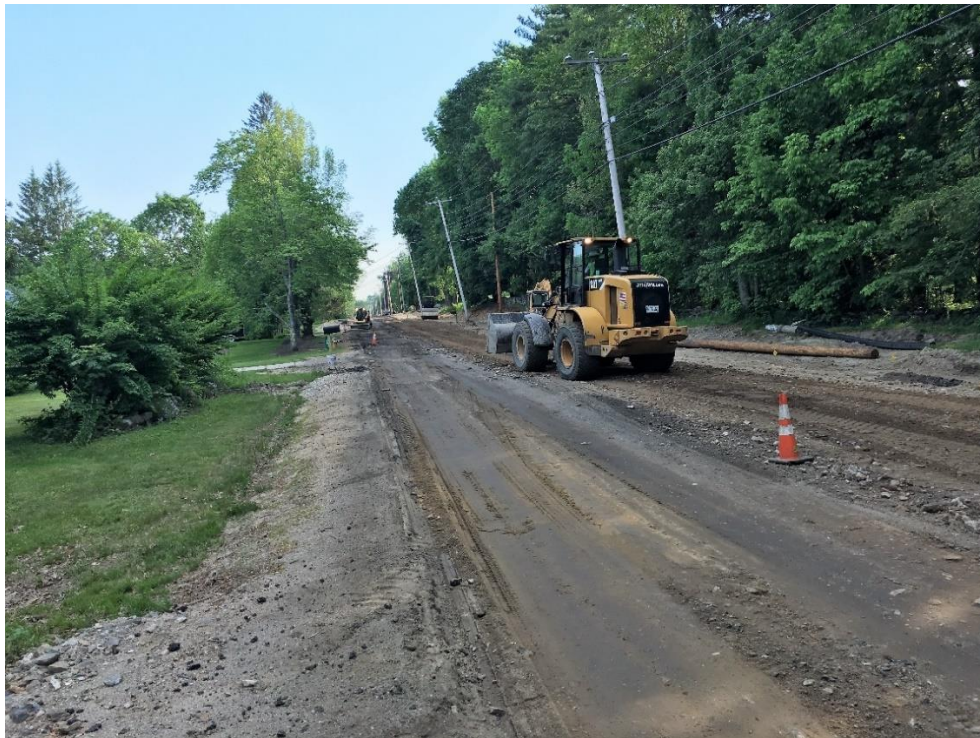
End of the day placement of temporary gravel to make road more passable after removal of pavement.
