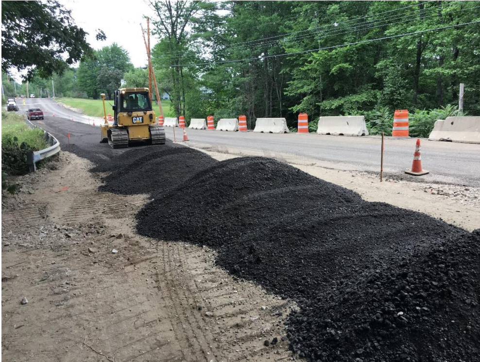
Began the day placing and compacting screened pavement millings over Type D subbase gravel in southbound lane from STA 57+50 southward.
