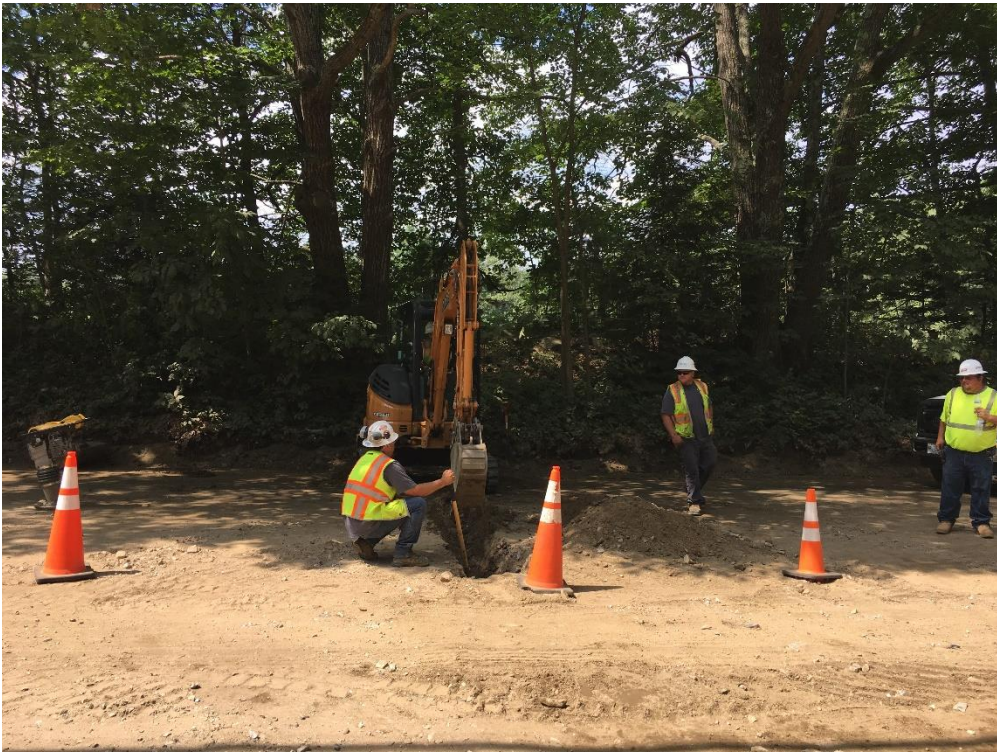
Summit trenching and installing PVC conduit sleeves across road for proposed "long side services."
