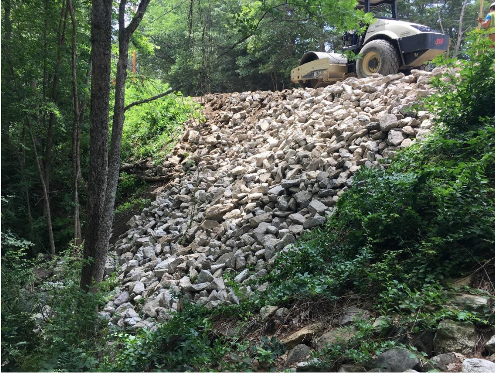
Placement of "Heavy Rip Rap" on outlet (east) side of Chernery Brook Gully above outlet of 42-inch culvert at STA 55+80.
