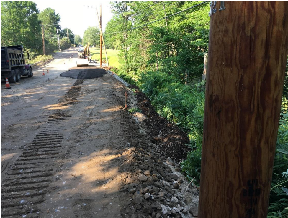
Placement of screened pavement millings (stable base for temporary jersey barriers) and erosion control mix along east side of road near steep slope in gully area.
