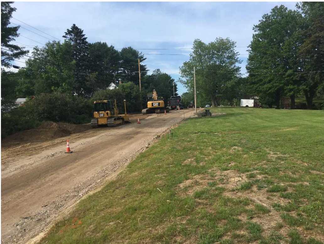
Finishing up the western side of the road prior to rolling near the end of the day.
