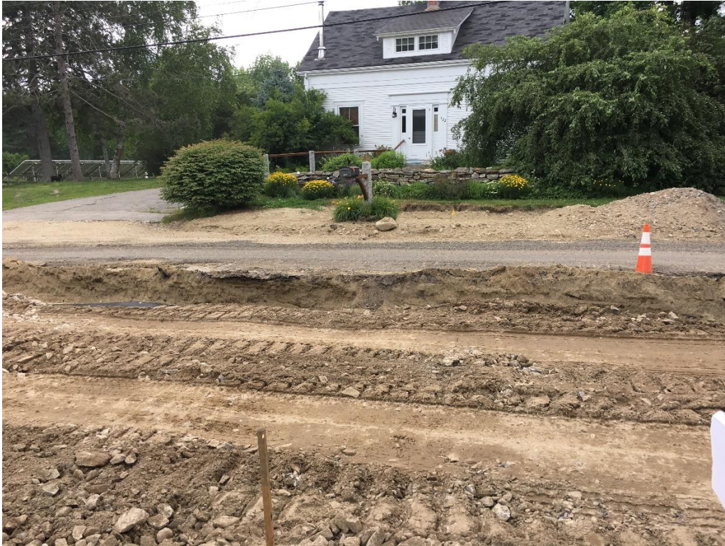
Completing the last 63 feet of full depth reconstruction from STA 61+12 to STA 61+75
