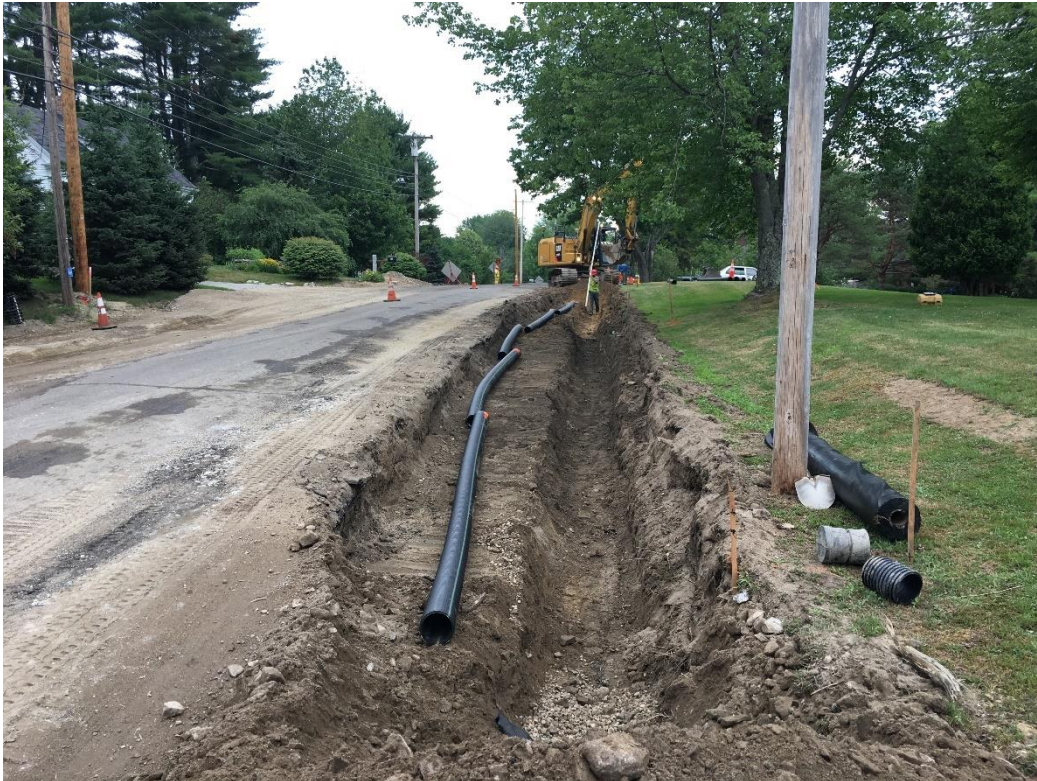
Completing the installation of 6-inch underdrain in east shoulder in front of Casey property.
