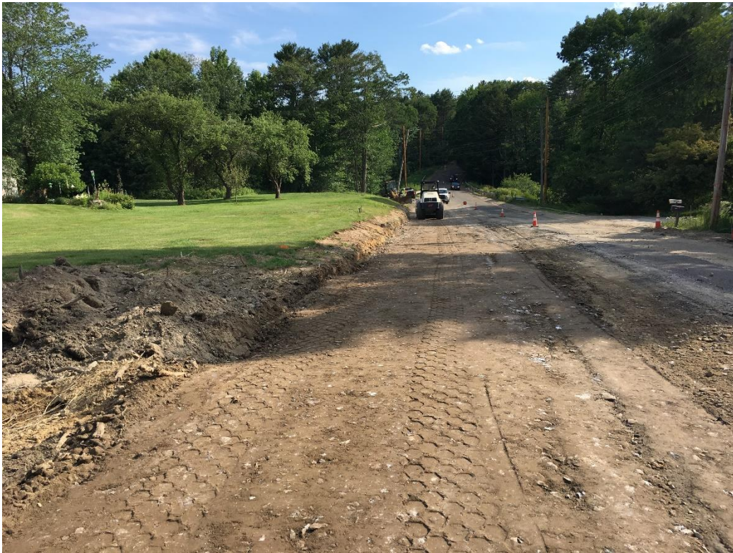
Compacting new gravel shoulder after installation of 6-inch underdrain at Casey property.
