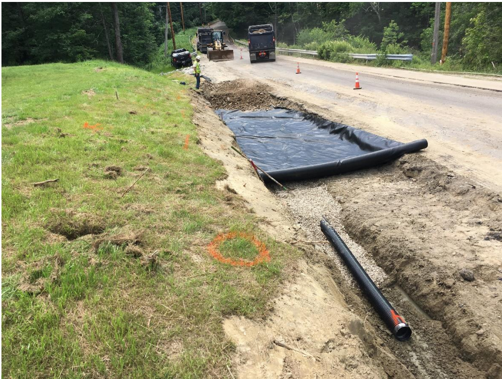
Installing 6-inch underdrain in shoulder just north of Cherney Brook in front of Casey property.
