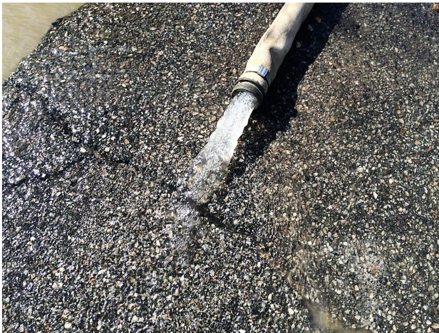
Discharge of trench dewatering after crushed stone sump installed.
