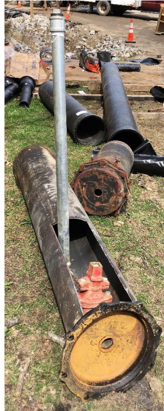
Blow-off valve assembly to be installed in Tuttle Road
