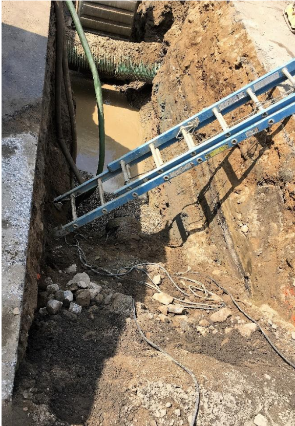
Water main connection trench in Tuttle Road to be installed under existing 18-inch sewer
