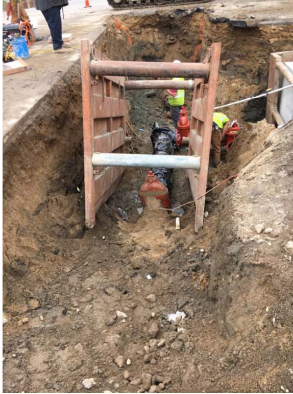
Installing 12"x8" tee on 12" line to Vault. Excavating existing 12" water main in Tuttle Road
