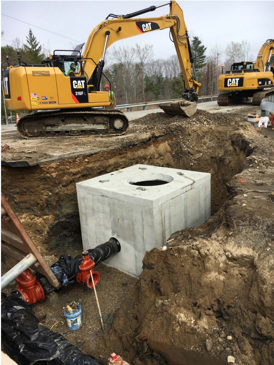
Backfill of vault underway
