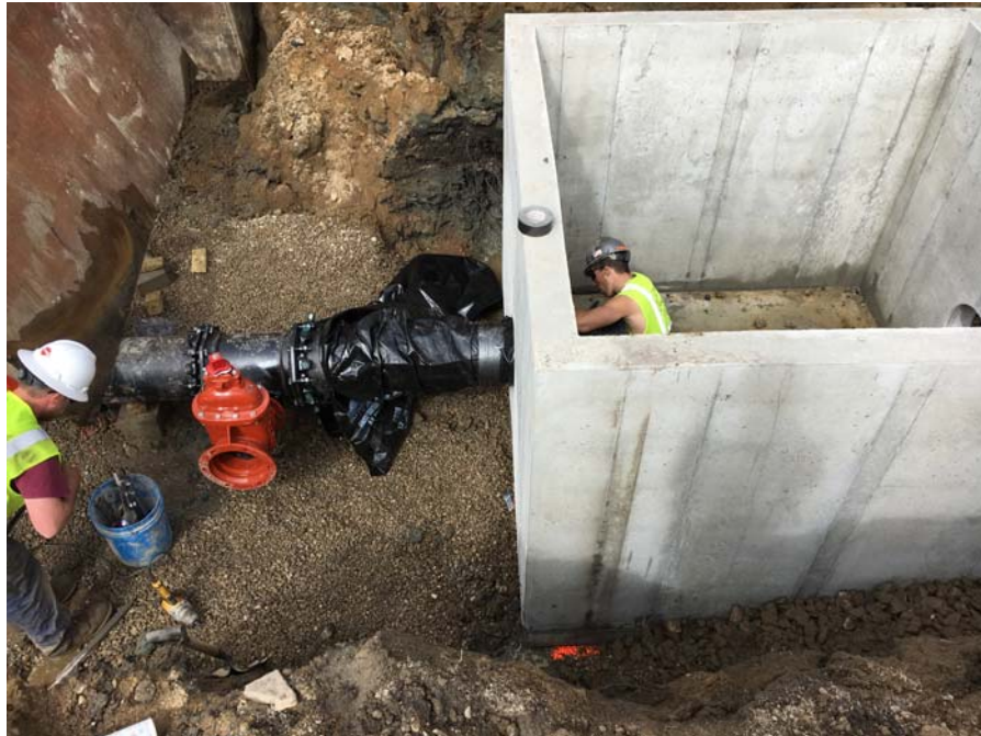
Connecting 12" water main to vault
