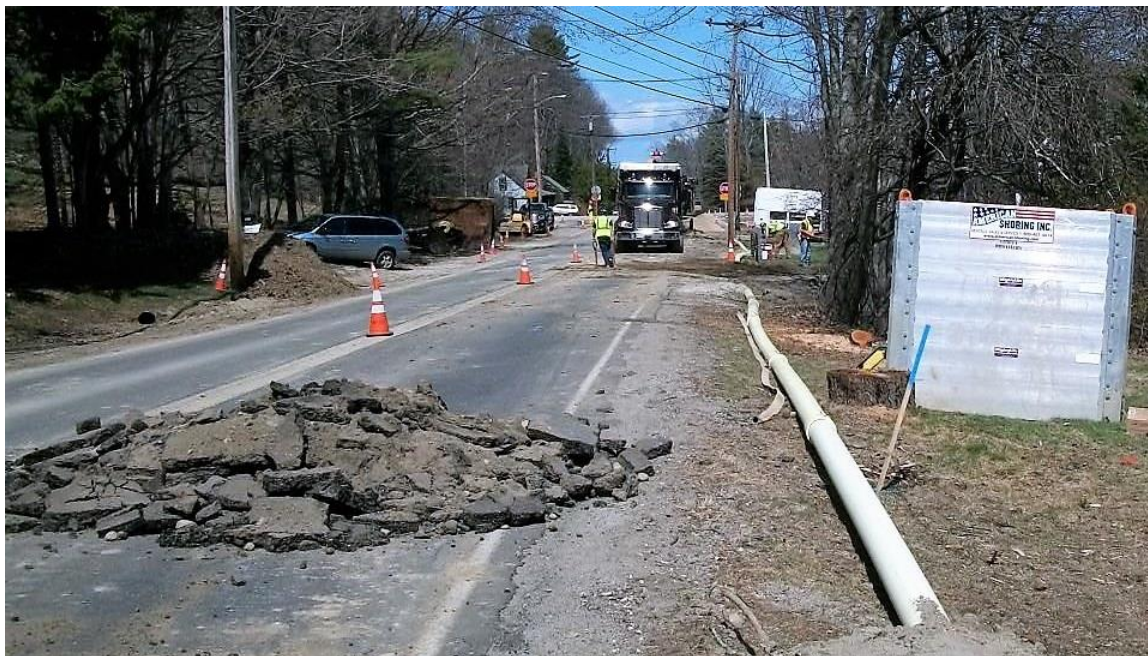
Temporary water main on east side of Middle Road looking north towards Tuttle Road.
