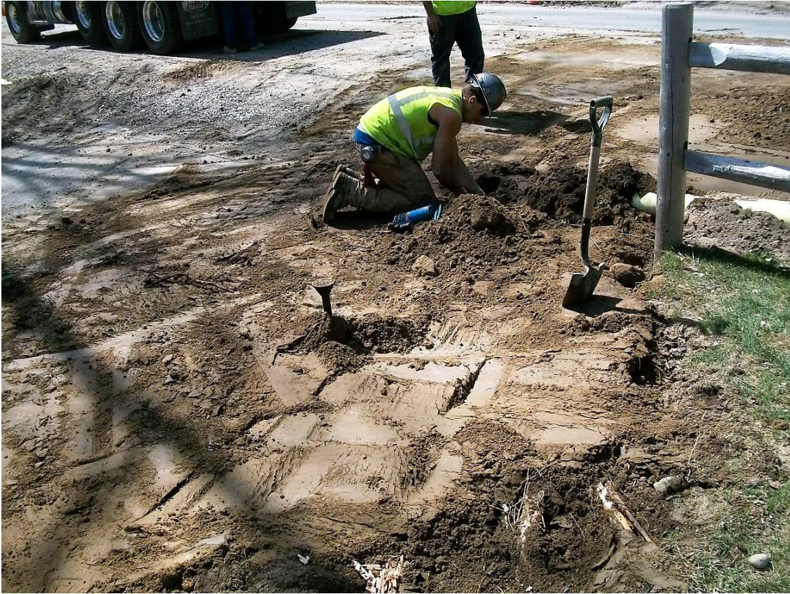
Installing a "renewed" service at 159 Middle Road (Byers) and reconnecting invisible fence.
