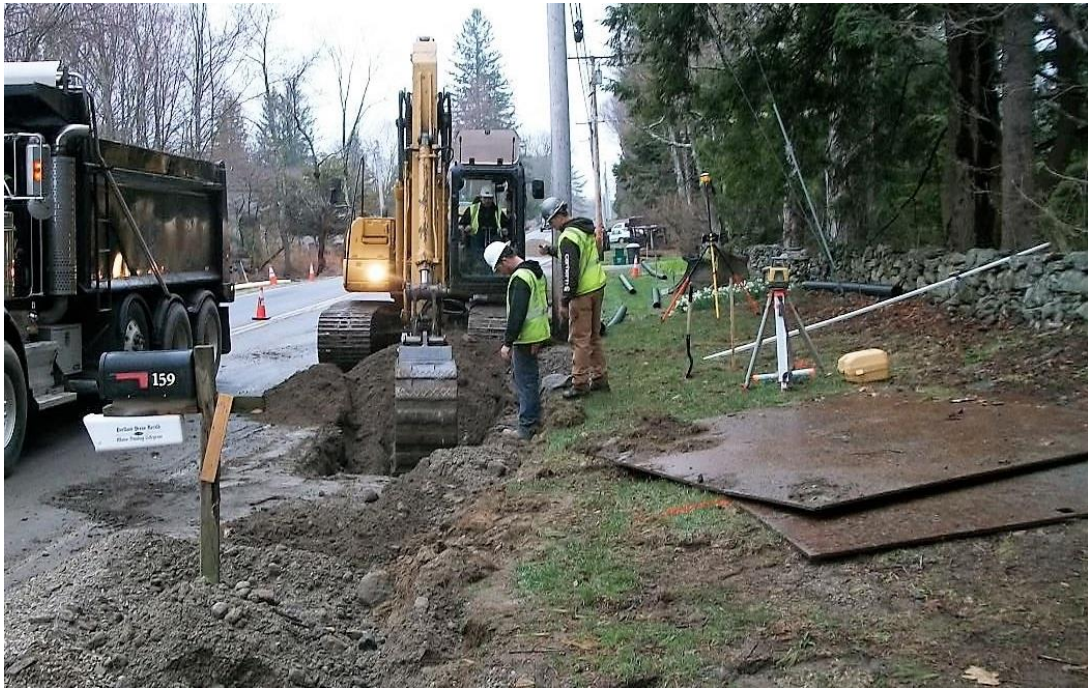
Excavation & installation of 6" underdrain uphill from CB-8B southward
