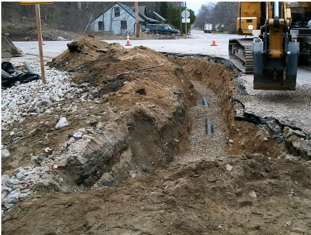
6-inch underdrain from CB-8A to Tuttle Road intersection
