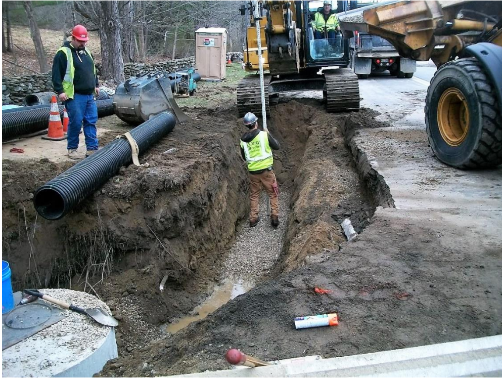
Trench preparation for new 12-inch underdrain from CB-8B (foreground) to CB-8A
