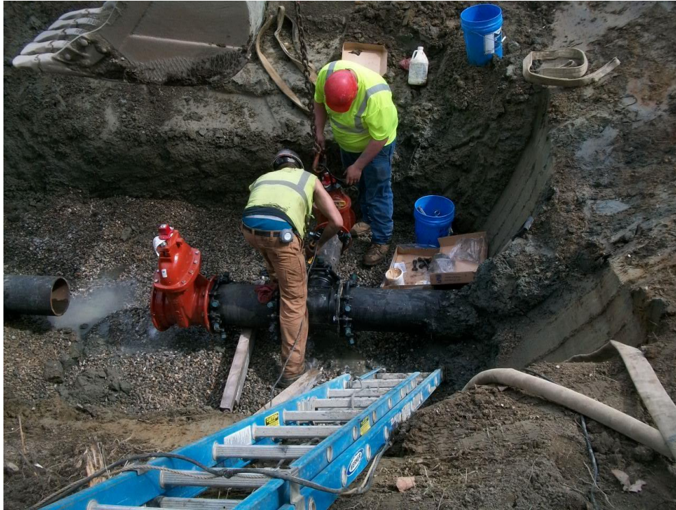
Cutting in gate valves south of Tuttle Road for temporary water main connections
