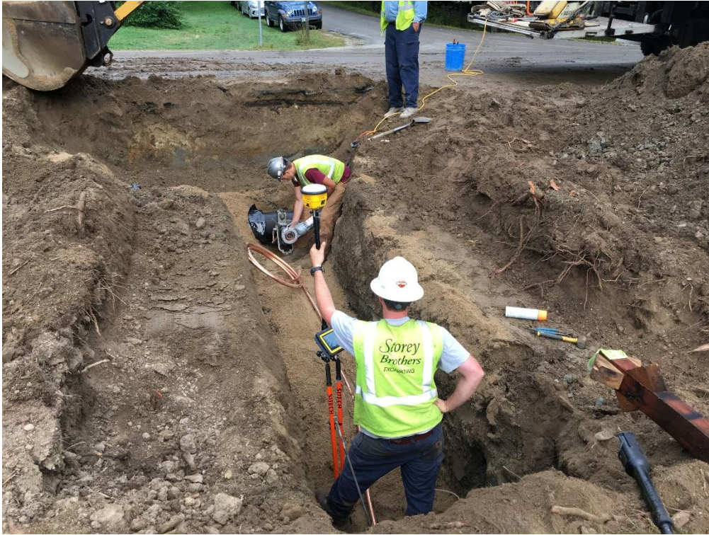
Tapping installed (but empty) section of water main extension for water service at 55 Middle Road near STA 27+60, RT (across the road from Rangeway).
