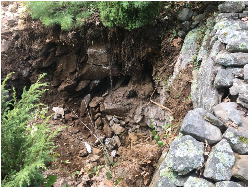
Additional ledge had to be broken up with a hoe ram attachment to excavator to install the final water service (at 72 Middle Road) near STA 36+60, LT.
