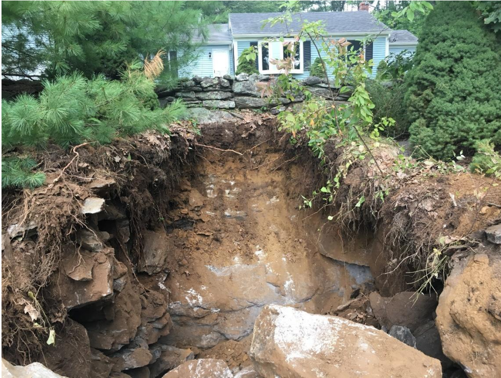
Steep ledge face at base of rock wall at 72 Middle Road. Crew to return the following day to install water service.
