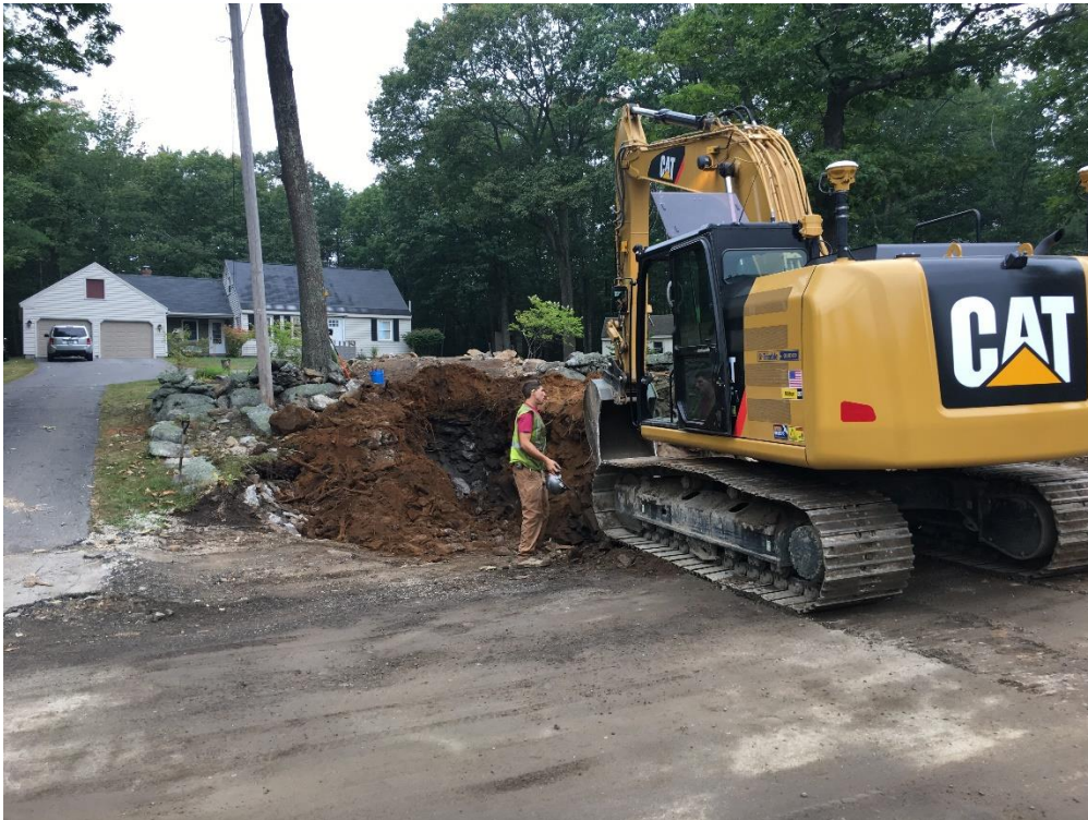
Installing "long side" water service at 70 Middle Road. Homeowner arranged with Contractor to have homeowner side blasted the previous week.
