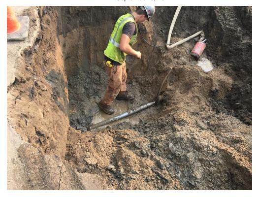
"Long side" services were mainly installed via the "Pneumatic Mole." Copper service line was pulled through the void which helped minimize traffic disruptions.
