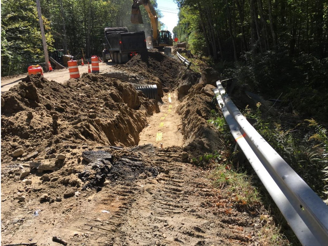
View of natural gas installation in sand bedding from the south with the warning tape above the pipe before installing the inlet section of the culvert.
