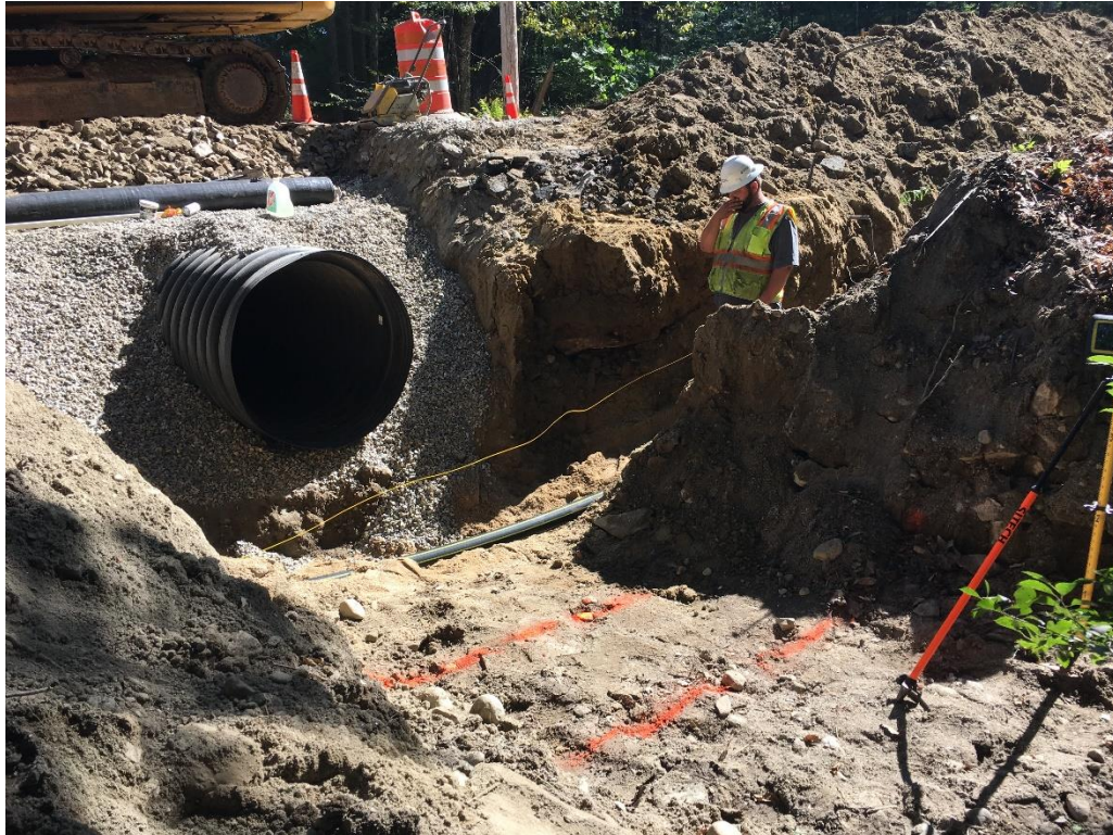
Installing 80-foot section of natural gas main under the culvert before installing the final section on the inlet side in the late afternoon.
