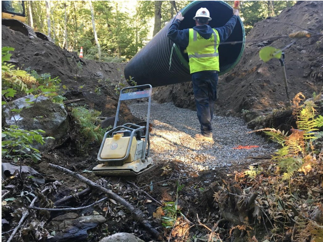
Placing the outlet section of culvert on compacted crushed stone bedding in the morning.
