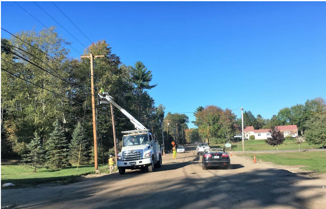
Transfer of communication lines onto new poles continuing north of the active work zone. This location is at Pole #311 at STA 40+12 in front of 80 Middle Road.
