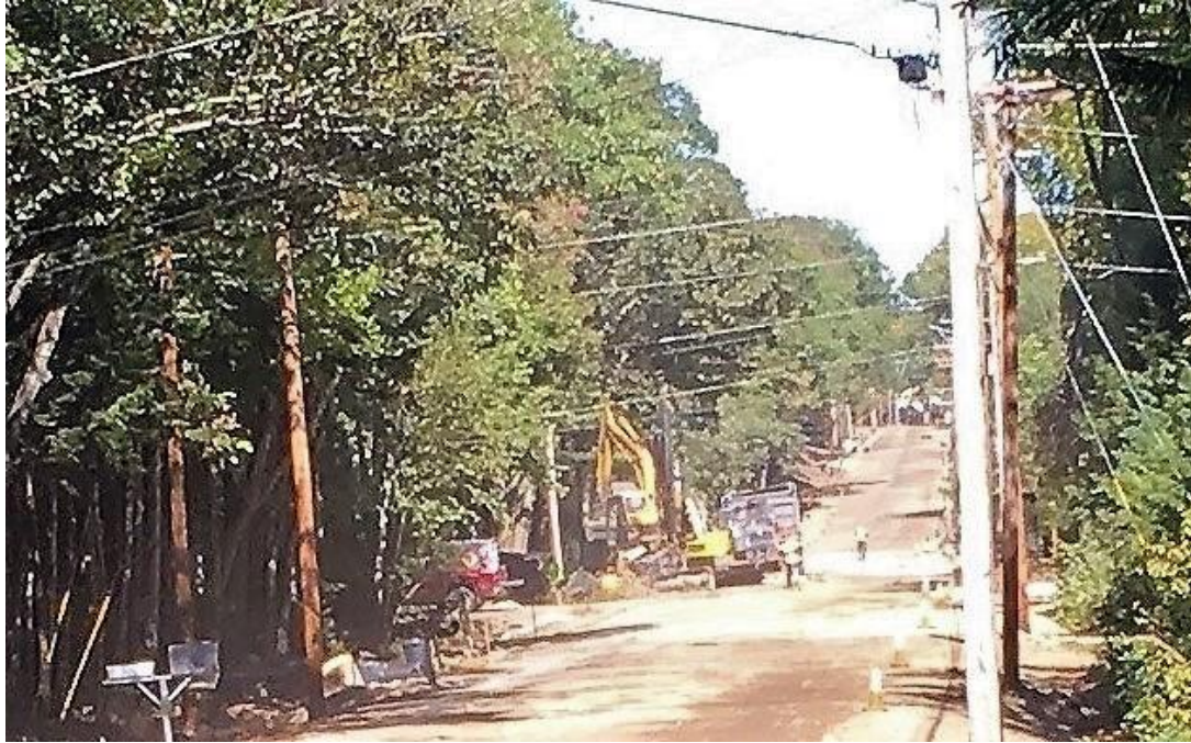
Blasting crew removing ledge for natural gas main in front of 44 Middle Road on west side of road about 700 north of water main installation on the east side of the road while a member of the Storey Brothers crew broadcasts calcium chloride on the road for dust control.
