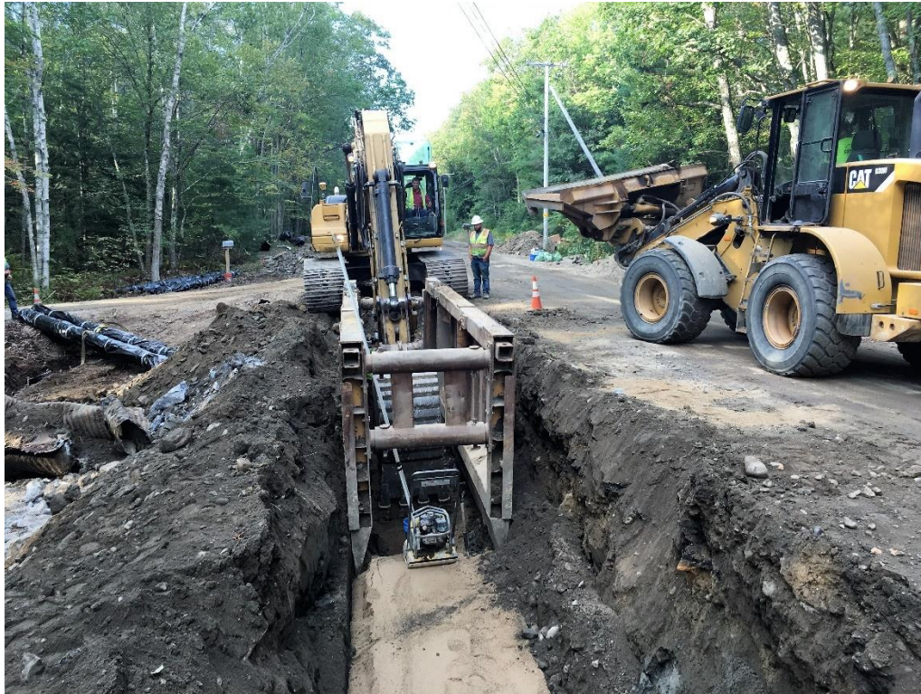
Preparing base of water line trench before placing bedding sand for next section of pipe.
