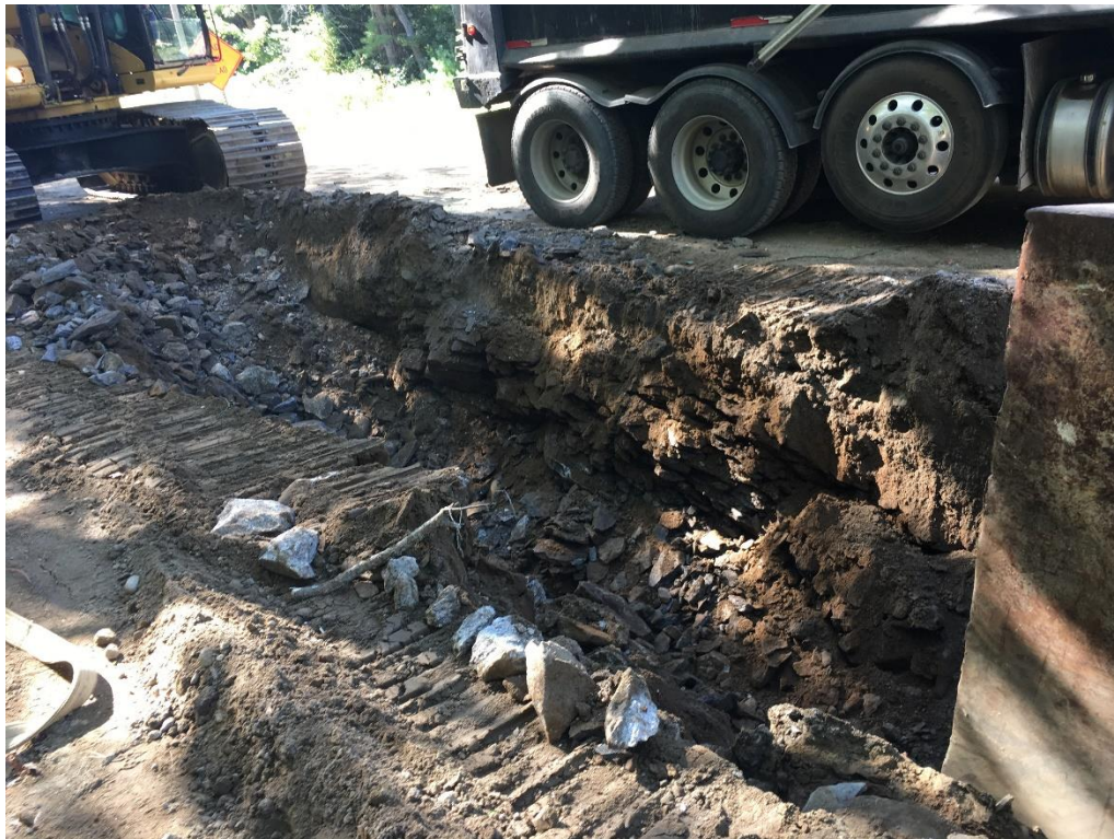
Profile of excavation ahead of trench box indicating ledge depth in the vicinity of Evergreen Lane.
