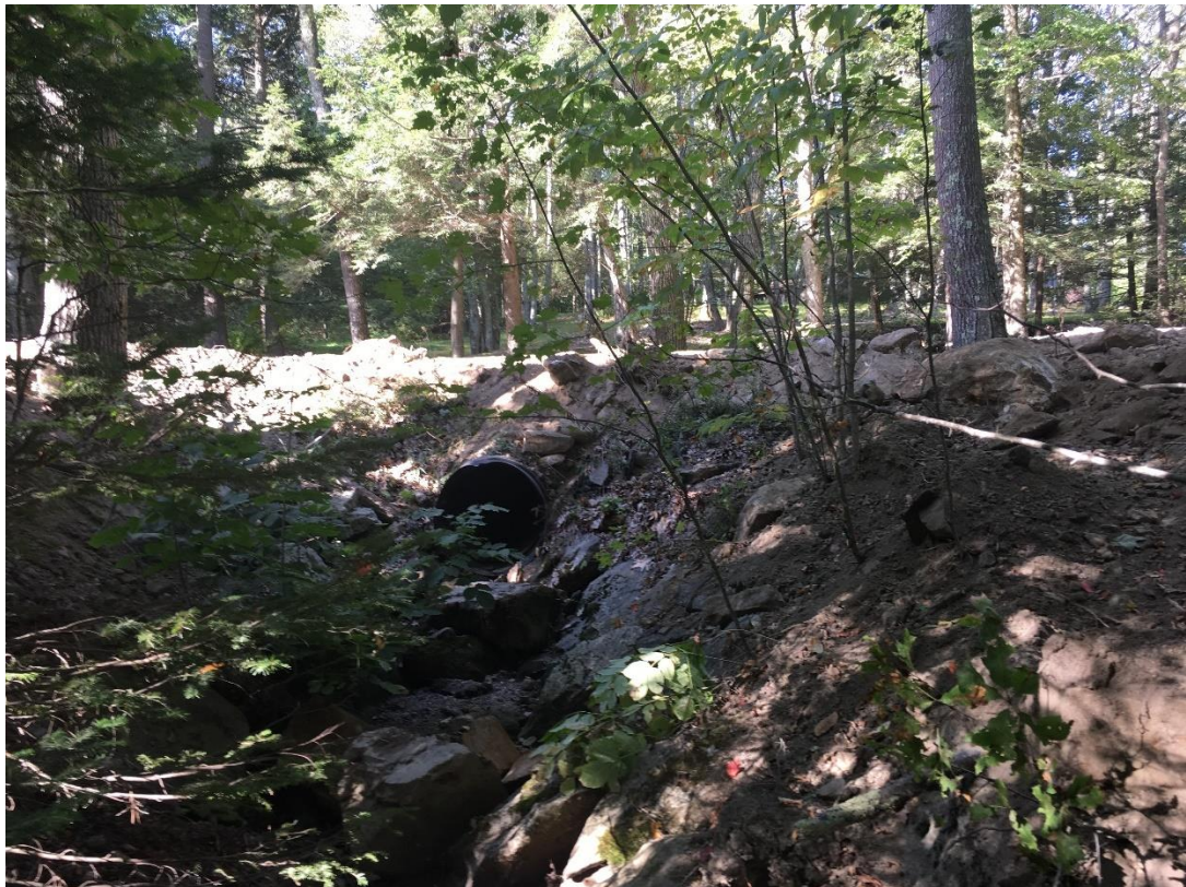
Unstabilized fill placed by owner of properties on Evergreen Lane in close proximity of the stream associated with the culvert crossing and retaining wall at STA 17+00.
