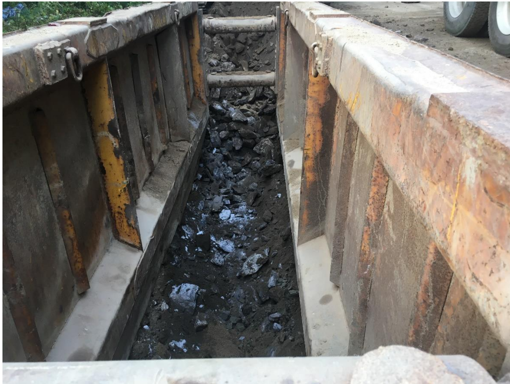
Dragging the trench box for the water main for the next length of pipe prior to excavating to final subgrade. Note blast spoils.
