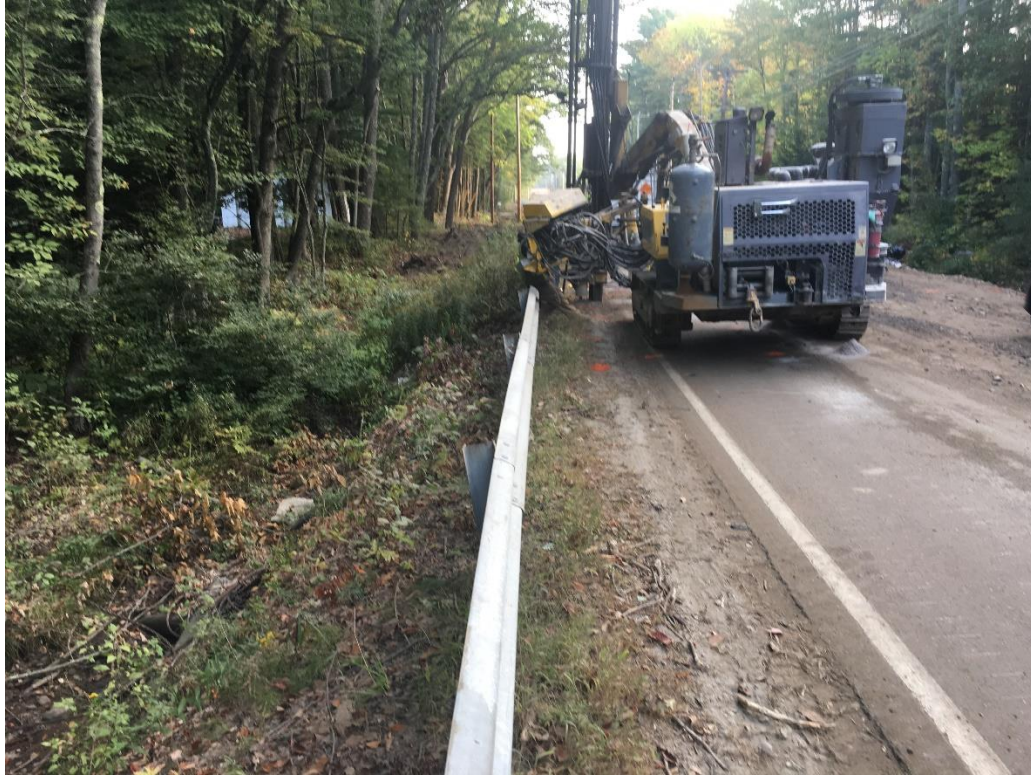
Drilling along the west side of the road at the culvert at STA 17+00 for the natural gas line.
