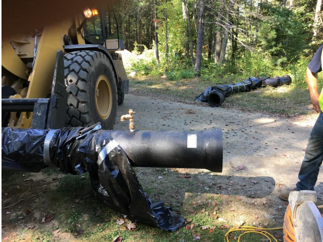
Water main tapped for 1-inch air release valve to be installed at STA 17+06 just north of "offset assembly." Offset assembly to go under culvert in background.
