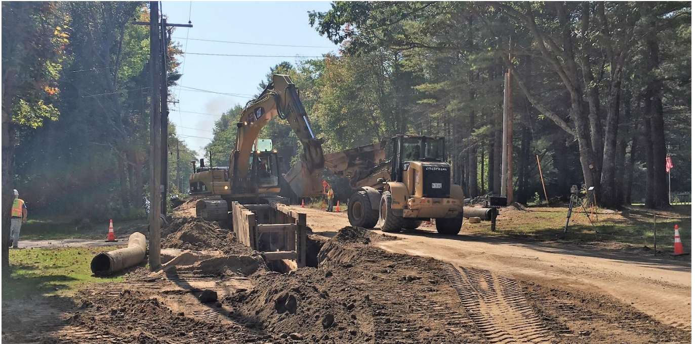
Backfilling the water line extension with sand delivered to the excavator by the loader with a "side dump bucket" near Shirley Lane.
