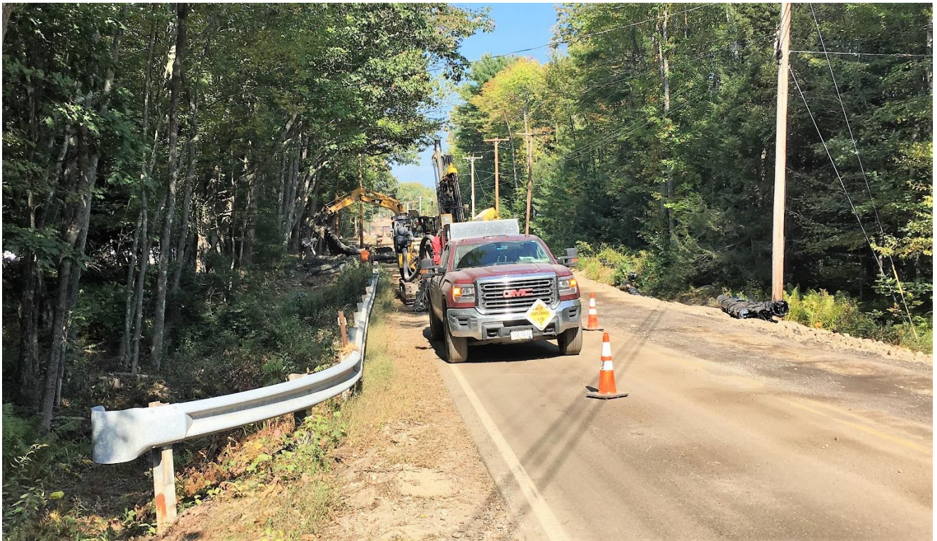
Placing the blasting mats prior to setting off a charge to remove ledge for a water service line at 34 Middle Road.
