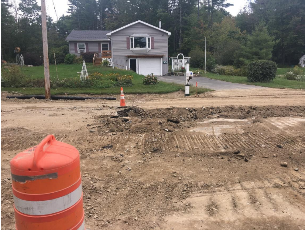
Matching up the east side box cut with the morning's west side box cut at the end of the day at STA 39+00.
