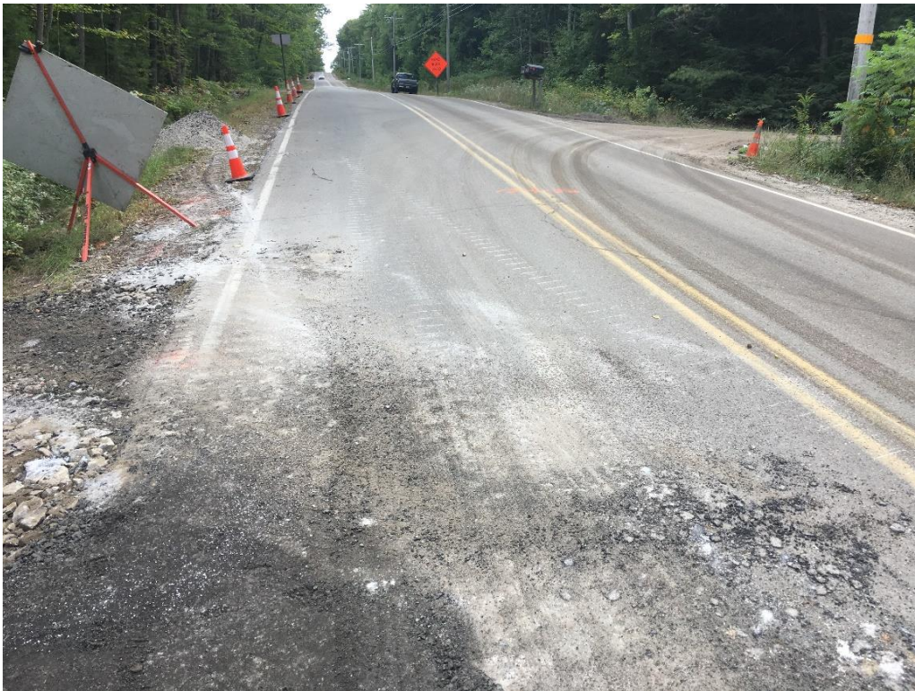
Clean up after the last blast of the day for water main extension at STA 15+75 just north of Evergreen Lane.
