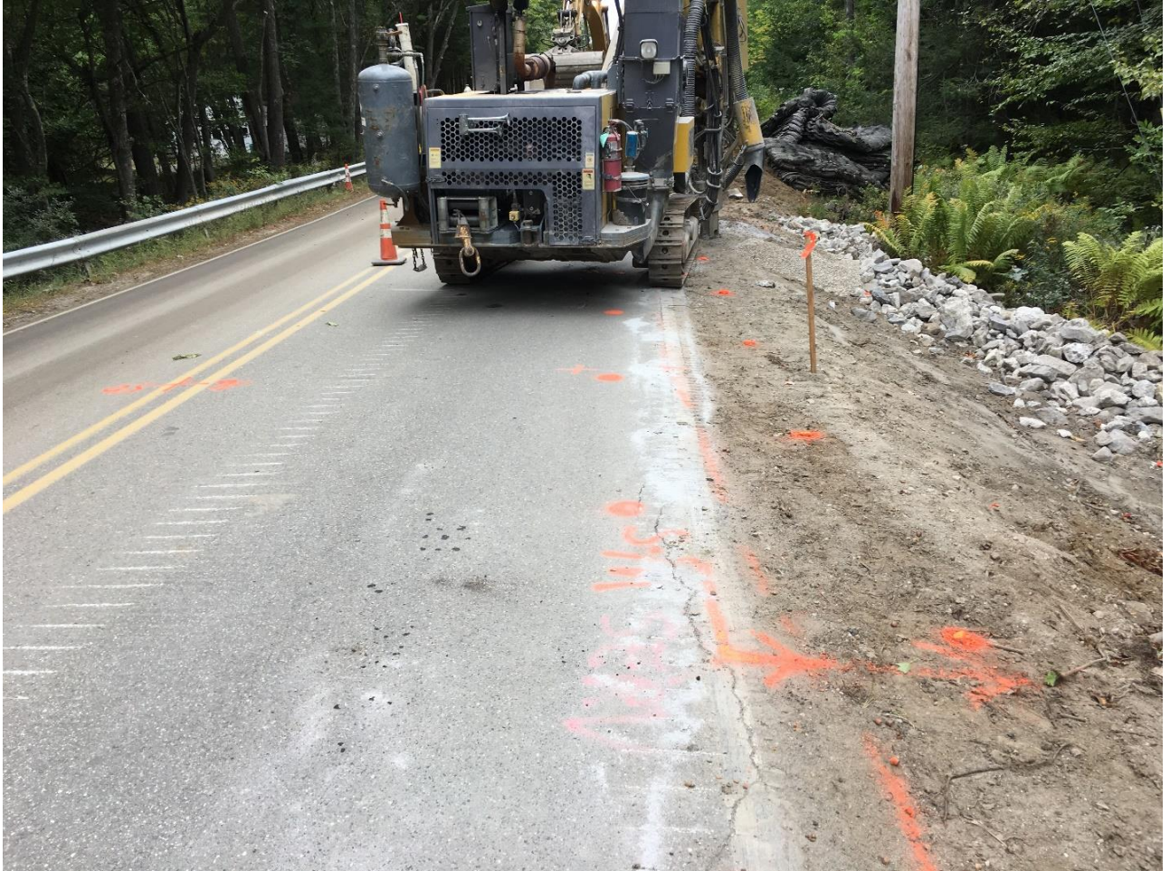
Blasting spacing south of the first blast of the day at the stream culvert at STA 17+00.
