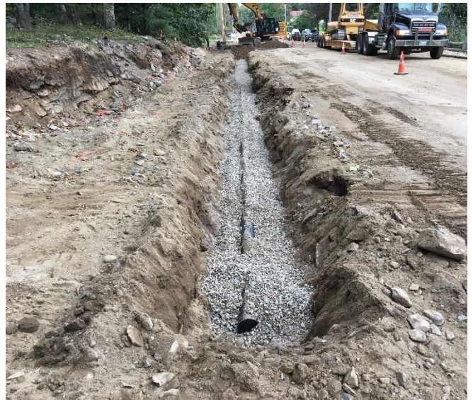
North outlet of underdrain installation on left at STA 39+70 and southern upland terminus of underdrain at STA 37+50. Total length is 220 feet.
