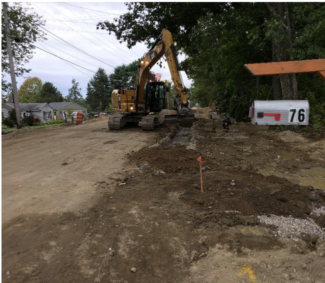
North outlet of underdrain installation on left at STA 39+70 and southern upland terminus of underdrain at STA 37+50. Total length is 220 feet.
